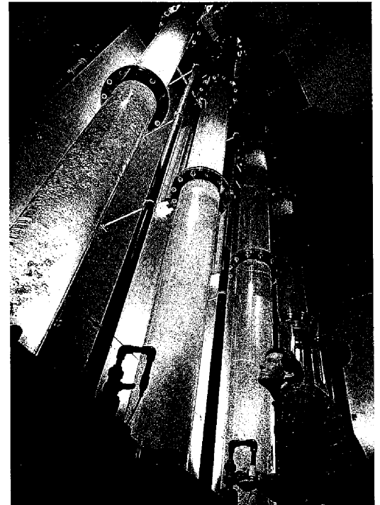
United Water pioneers water and wastewater treatment through innovative technologies such as ozone treatment, an advanced drinking water purification process. United Water, which operates a state-of-the-art ozone plant in New Jersey, is evaluating the ozone process in New York.
