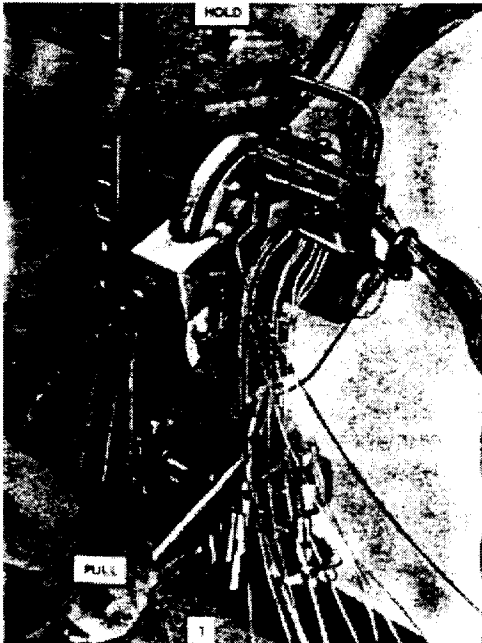
Fig. 35—Seating and Cutting conductors
