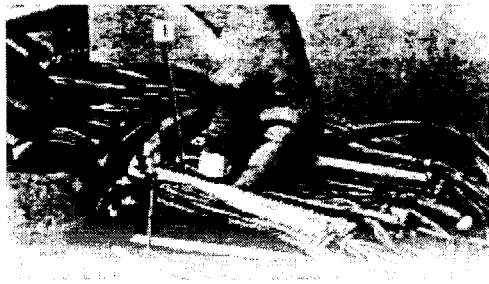
Fig. 178—Placing Cap on Bridge Module
