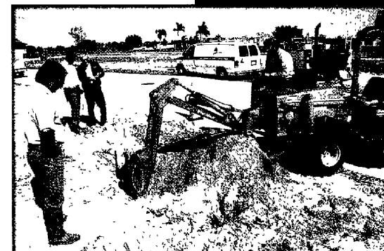
Repairing A Gas Main In West Palm Beach
