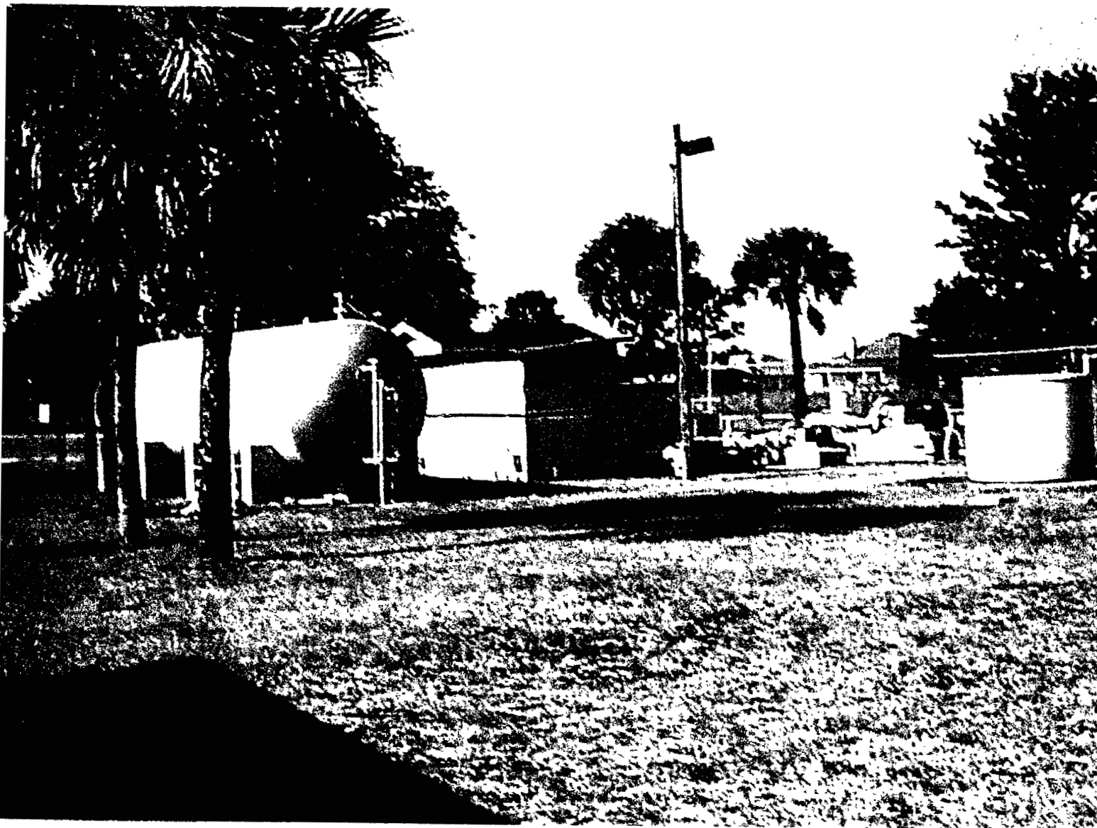
VIEW OF TREATMENT FACILITIES
