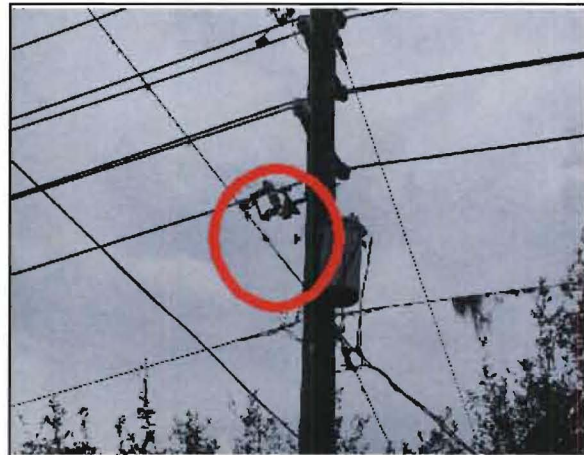
Sobrino No. 6: Pole is located at the intersection of Magnolia St. and 6th Ave., north on CR 435 and west on CR 439 towards Windermere. Failed lightning arrester.
