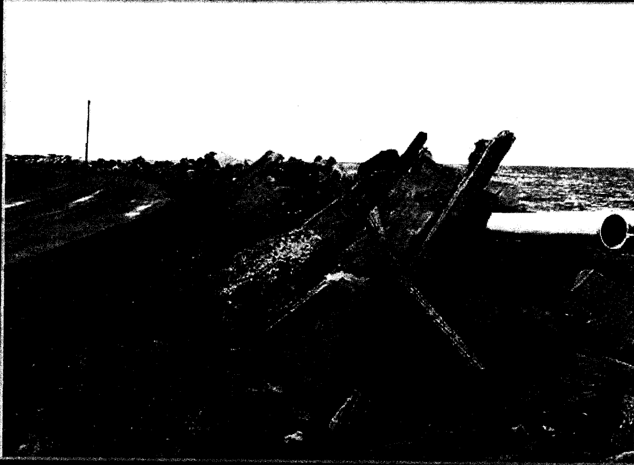
Alligator Pt: 600 pair cable uncovered and cut by storm
