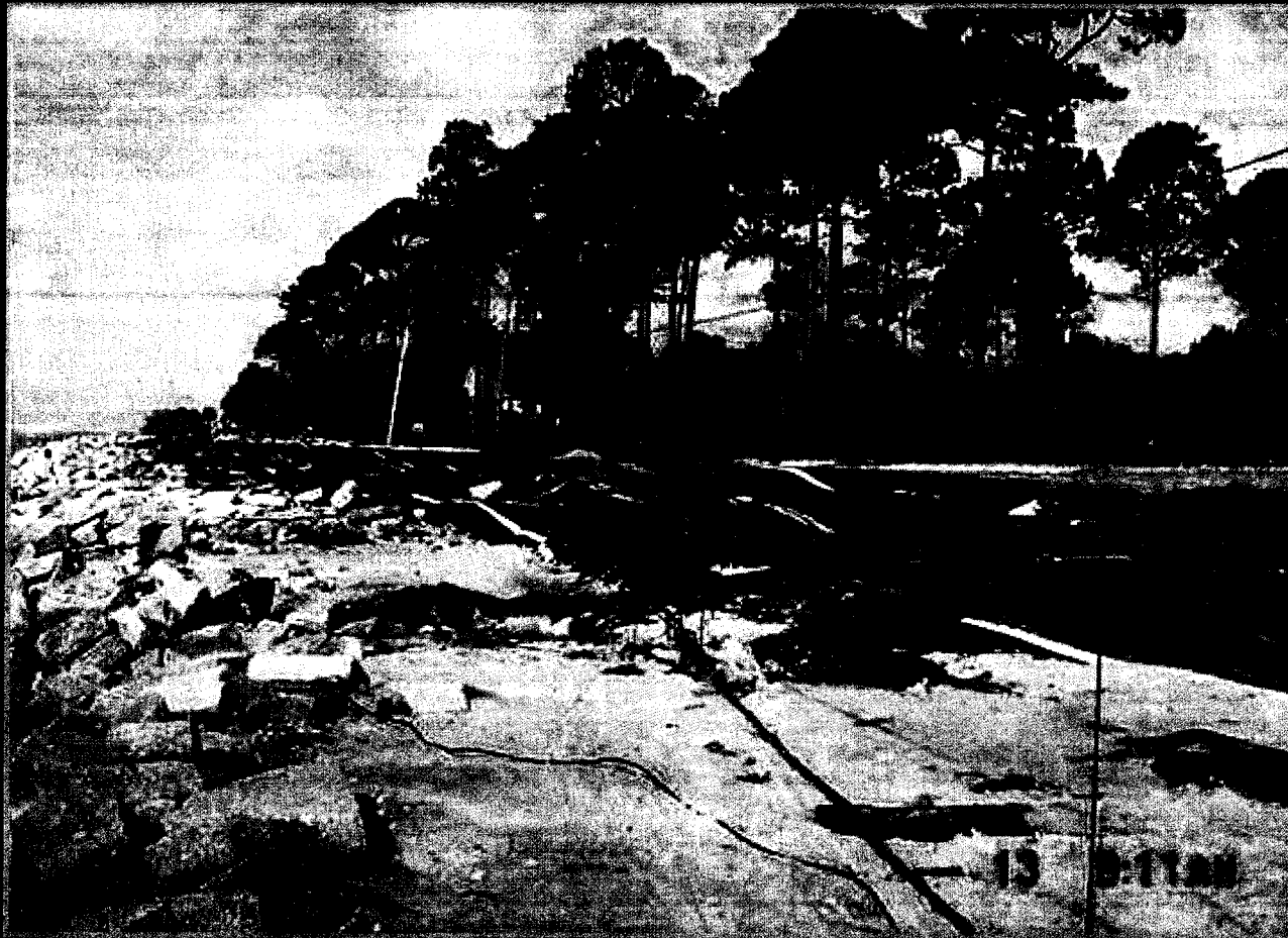
Carrabelle Bch: Fiber and 100 pair cable torn all to pieces
