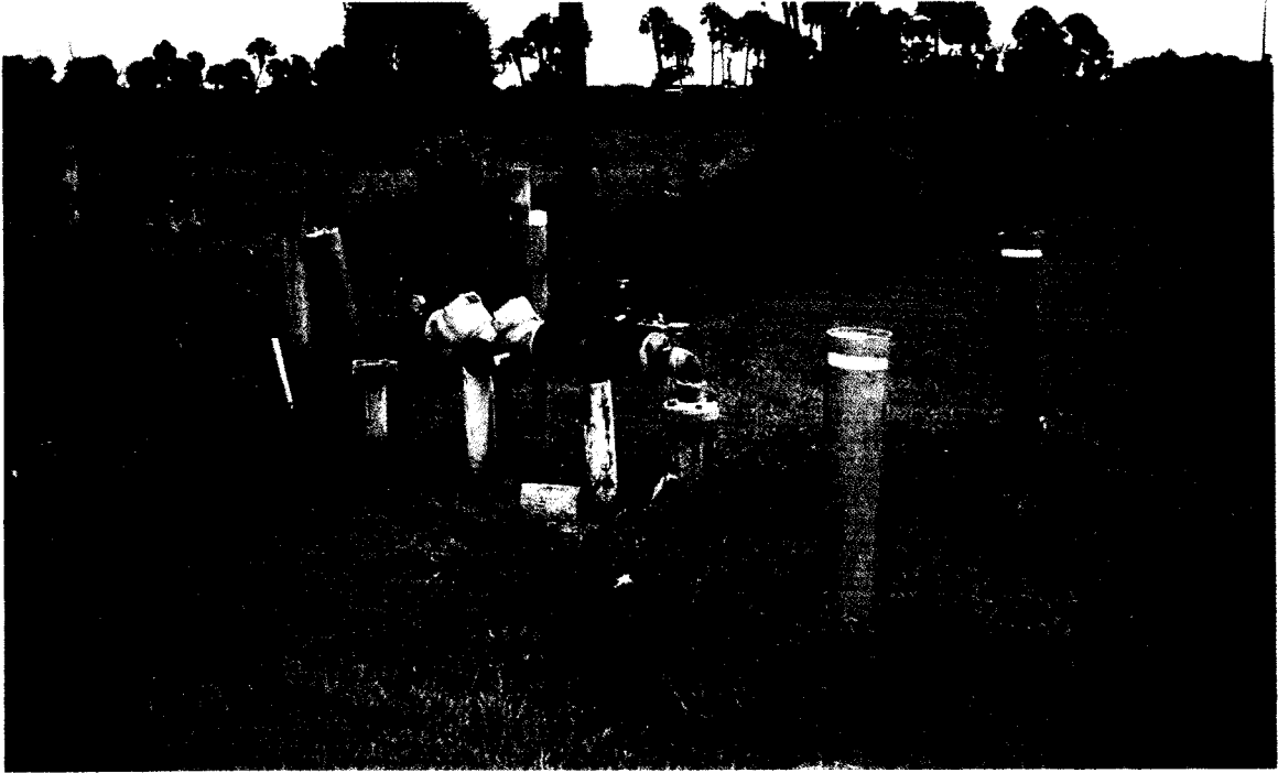
Connection to Seminole Water Plant
