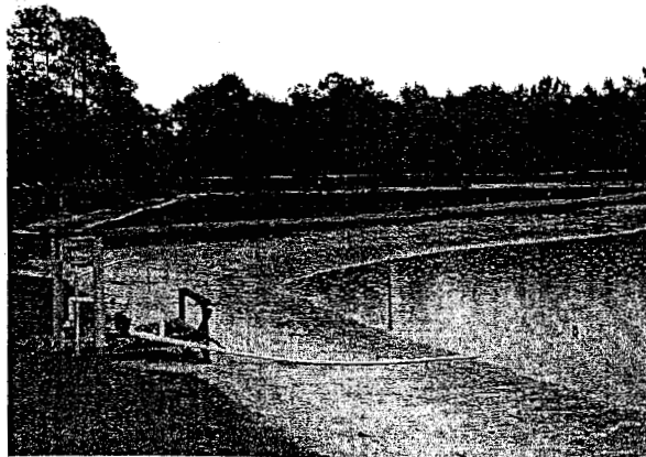
Evaporation Ponds : 2 Far Basin: Effluent Holding Pond for Evap. Pond Near Basin: Evap. Pond via Pumping to Sprinkler Heads
