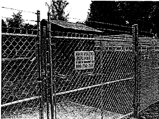
WWTF Grounds: Fenced & Secure
