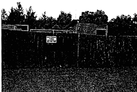
WWTF Perimeter Fence : Weathered Wood Fence Requiring Reinforcement / Replacement
