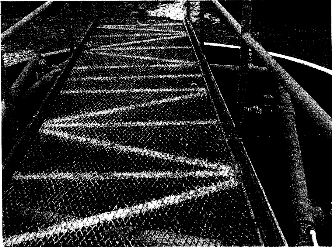
Photo #2: Holes in grating over treatment plant.
