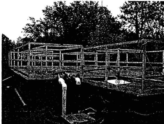
WWTF: Lift Station
