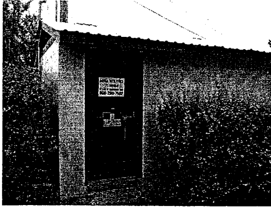
Off-Site Master Lift Station
