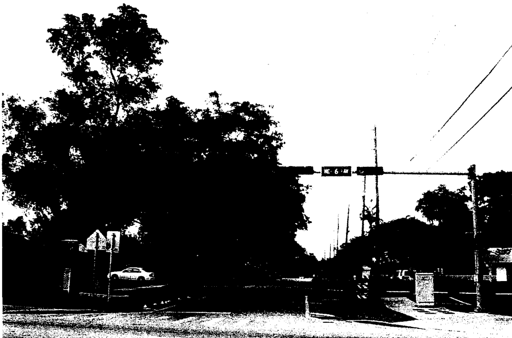
5 6 Photo 6: Looking west from the corner of NE 6 Avenue and NE 107 Street, the north side 7 of the street has a 3 phase feeder line, with only smaller maturing trees planted under the 8 lines (a Crape Myrtle is under the lines). The south side of the street is planted with Black 9 Olive trees that provide canopy and shade to the road and properties. This is an example 10 of good planning for continued utility reliability based on keeping trees outside a 11 potential conflict with the overhead lines. 12
