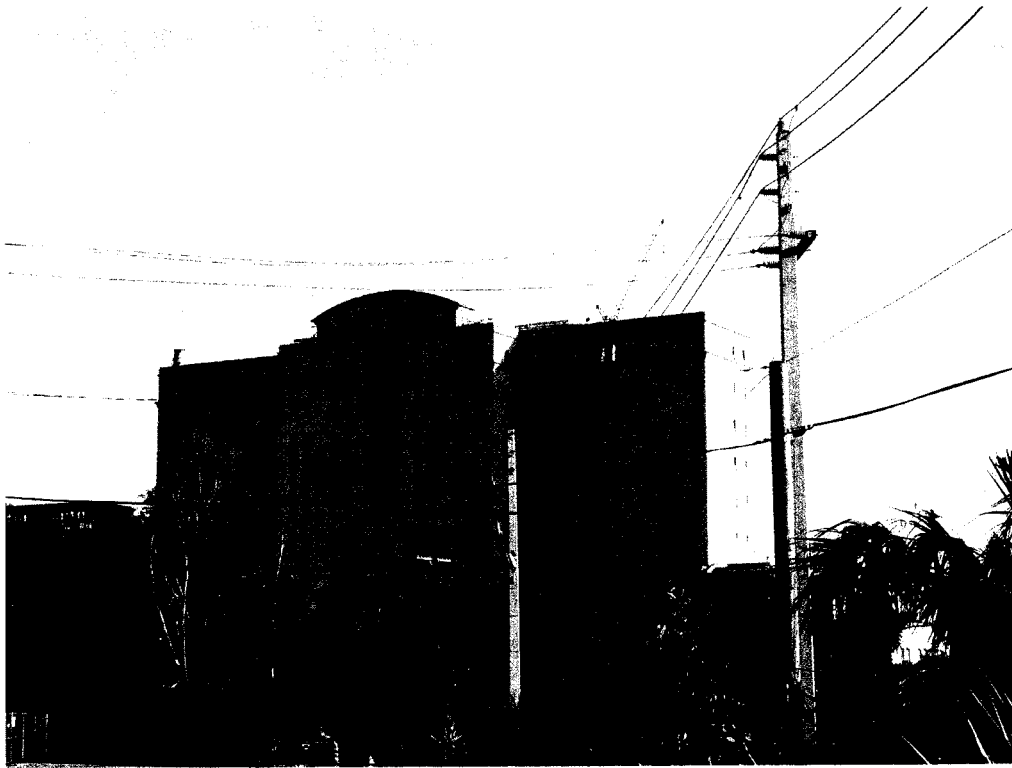
CIF Feeder serving VA Hospital in Palm Beach County hardened to EWL
