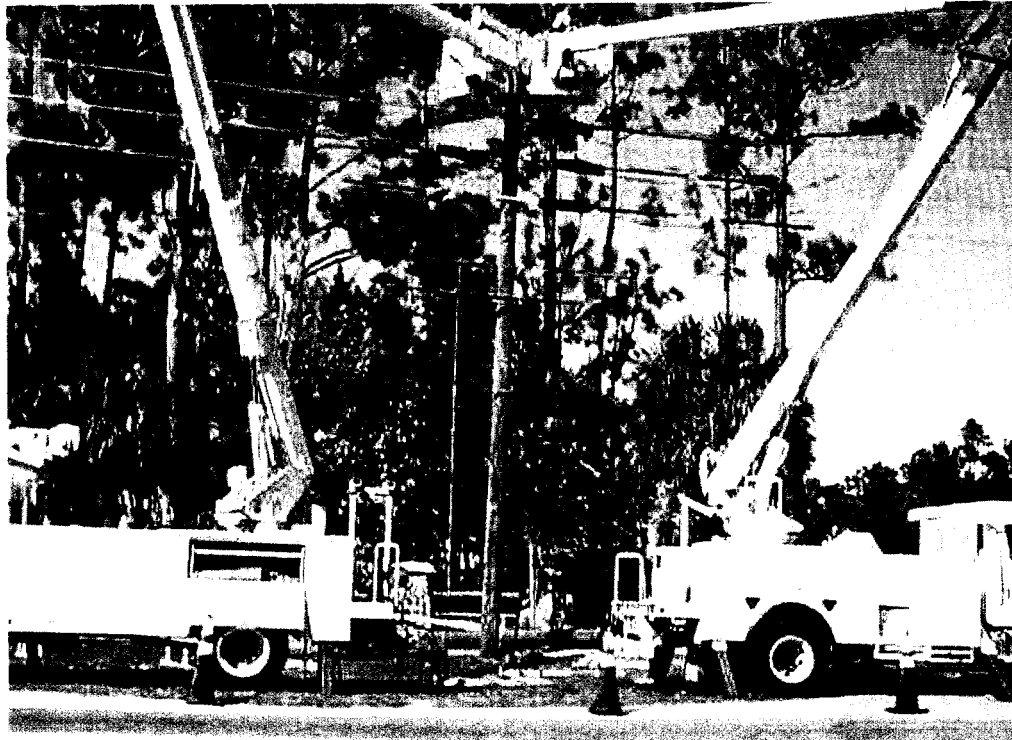
EWL hardening CIF Feeder serving Halifax Hospital in Central Florida
