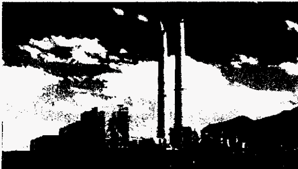
PacifiCorp's Huntington Power Plant in Huntington, Utah
