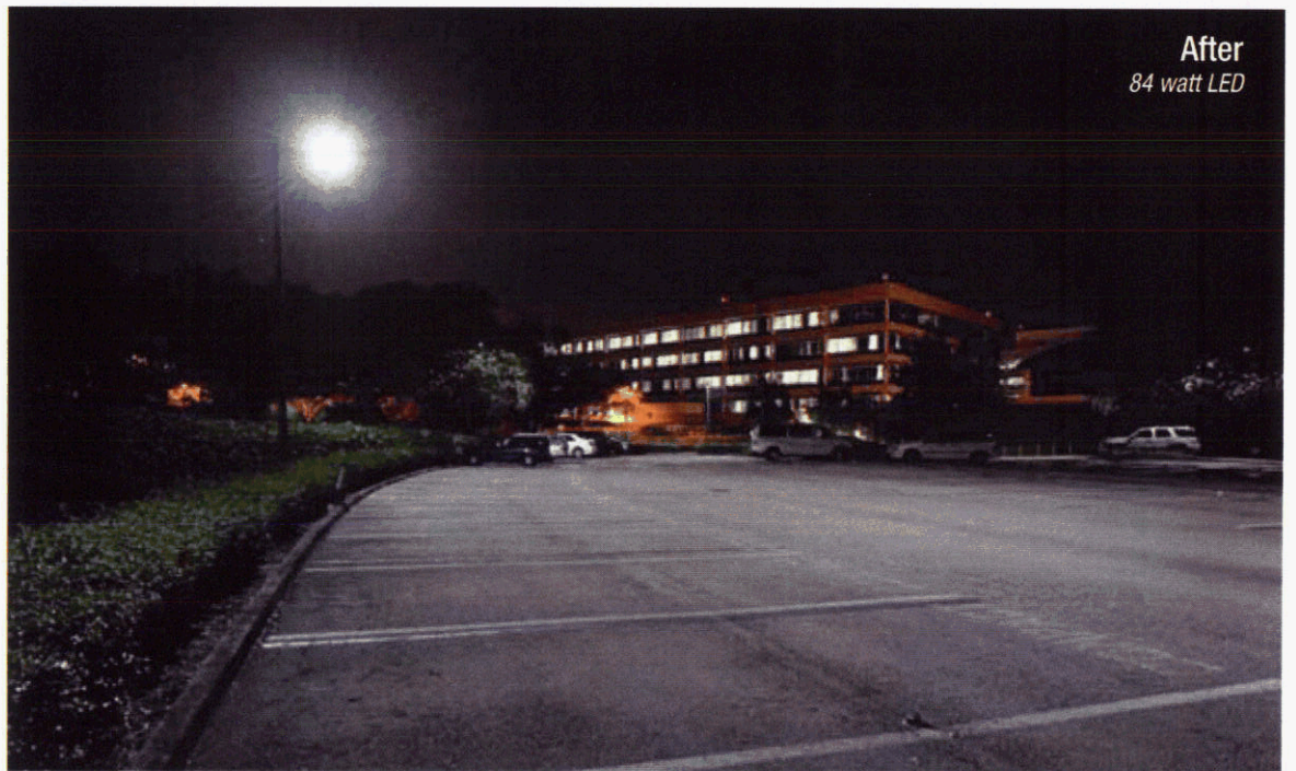
Before 250 watt HPSV
