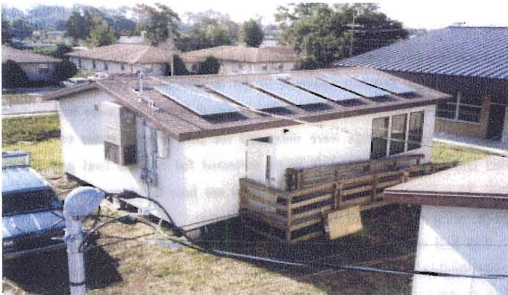
Figure 4-2 Portable Classroom Topped by PV Panels
