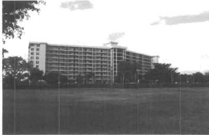
Palm Aire Condos FPL Roof Coating, 8 Buildings - Pompano Beach, FL
