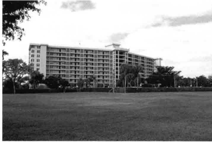
Palm Aire Condos FPL Roof Coating, 8 Buildings - Pompano Beach, FL
