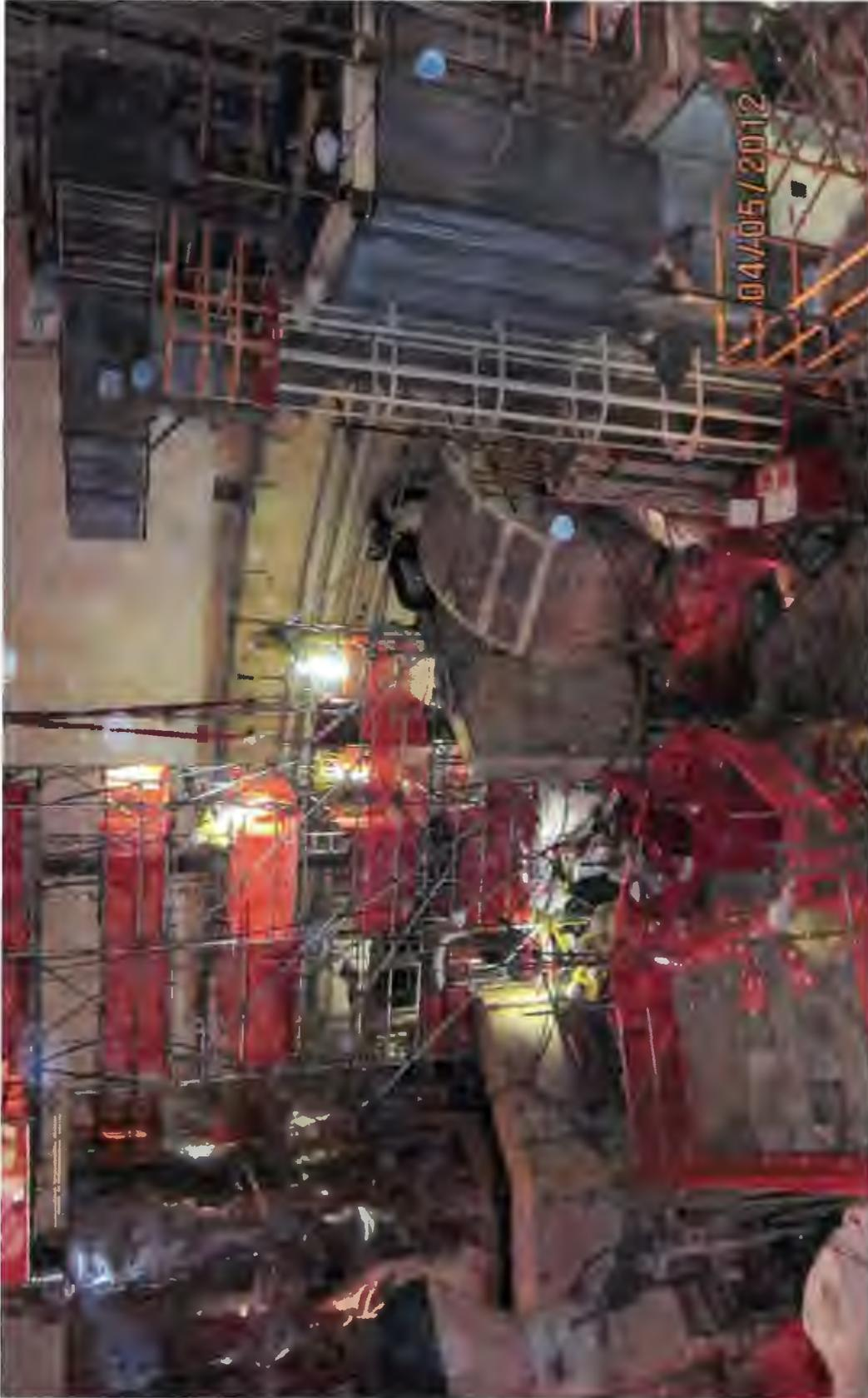
Primary Containment with scaffolding being erected to support crane erection and access for workers.
