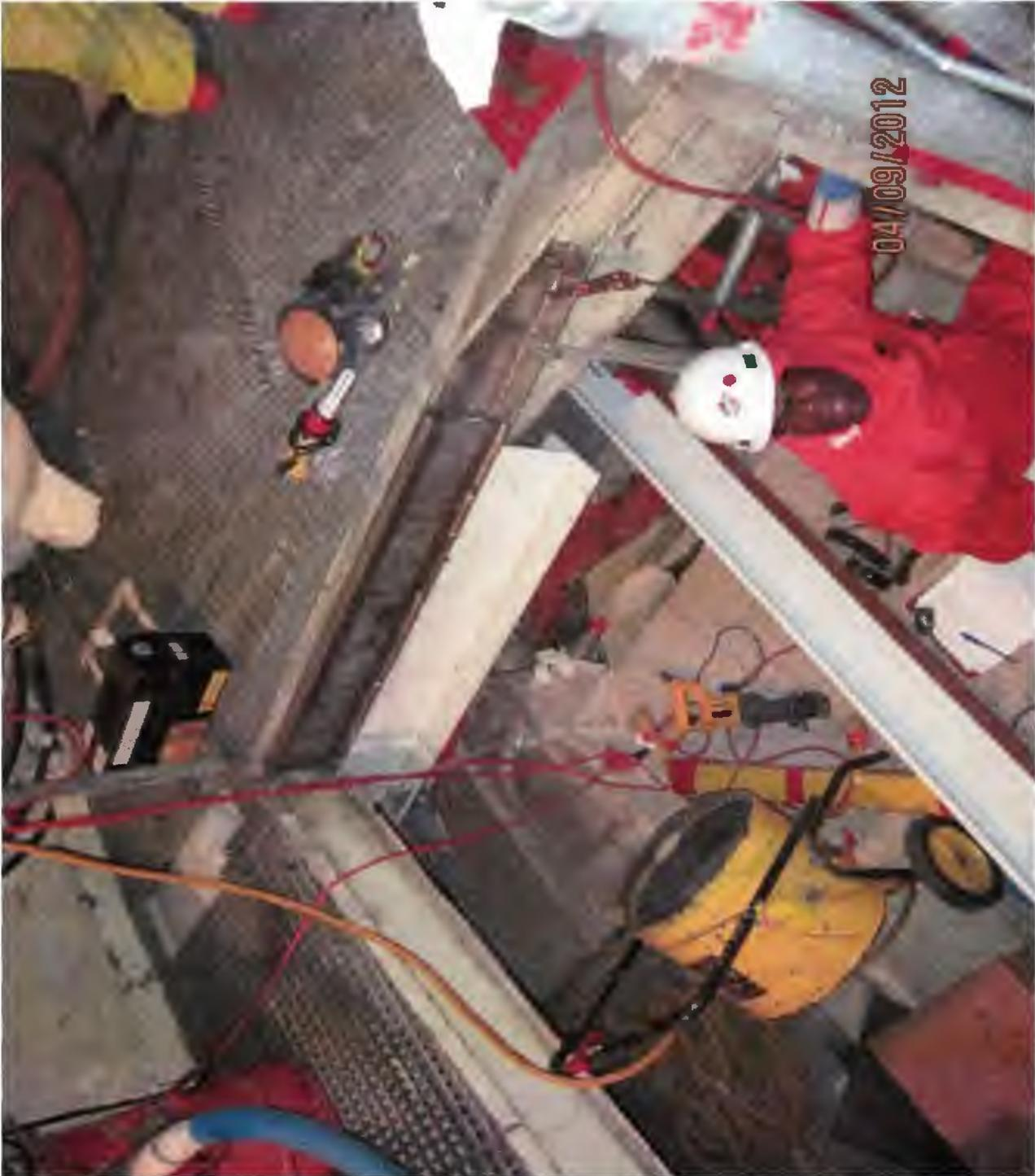
Primary Containment. Worker in protective clothing adding structural material in support of the Normal Containment Cooler modification.
