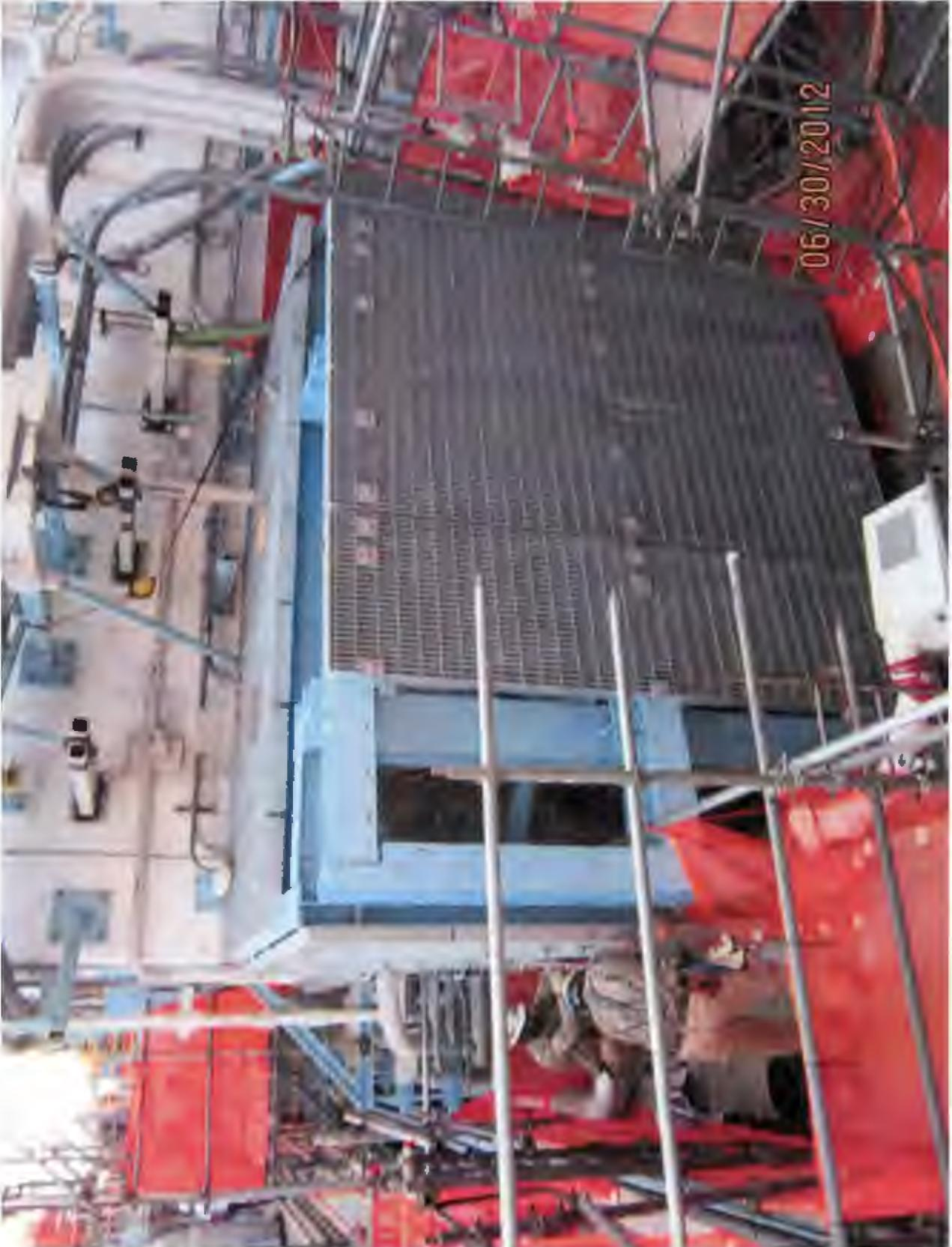
Turkey Point. Workers complete the installation of the missile barrier structure for the CREVS/CREFS systems.
