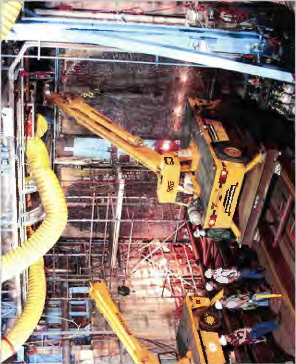
As part of the condenser upgrades, workers removed legacy tube sheets using acetylene torches to simultaneously cut and remove both sheets from all condenser bays. Like many EPU modifications at Turkey Point, the removal of the tube sheets was a first-time evolution, thus requiring careful planning and execution.
