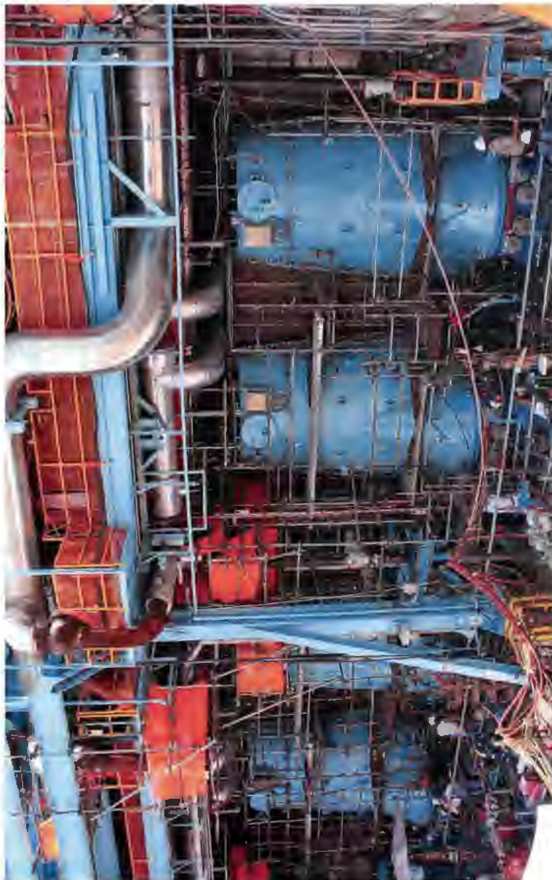
The condenser blue water boxes complete the condenser tube bundle replacement. The water boxes receive the canal cooling water leaving the more than 55,000 new condenser tubes and directs the cooling water to the discharge piping which returns it to the cooling canal.
