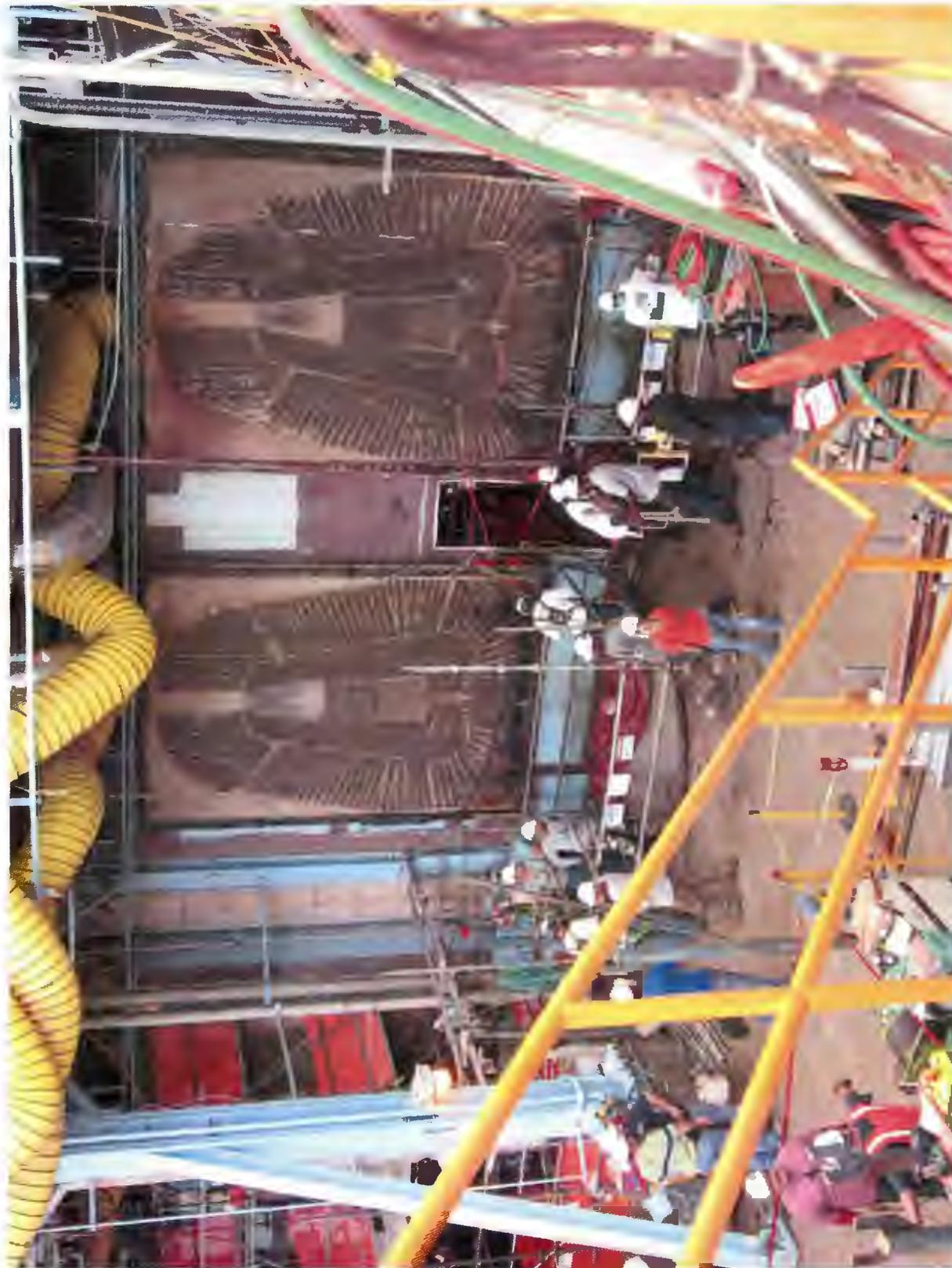
Turkey Point main condenser tube sheet plate which holds the cooling water tubes in place. These are removed and the new condenser tube bundles are installed
