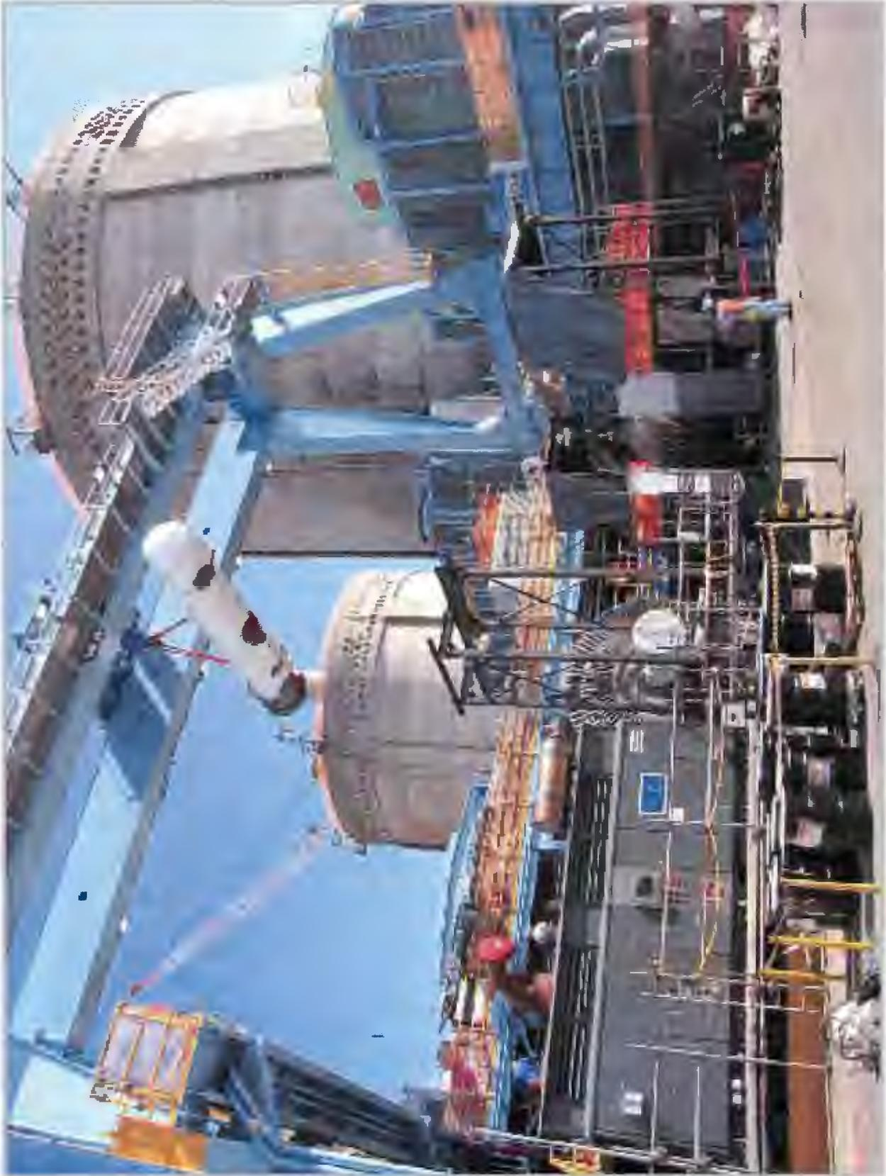
One of four feedwater heaters lifted from the staging area to the turbine deck.
