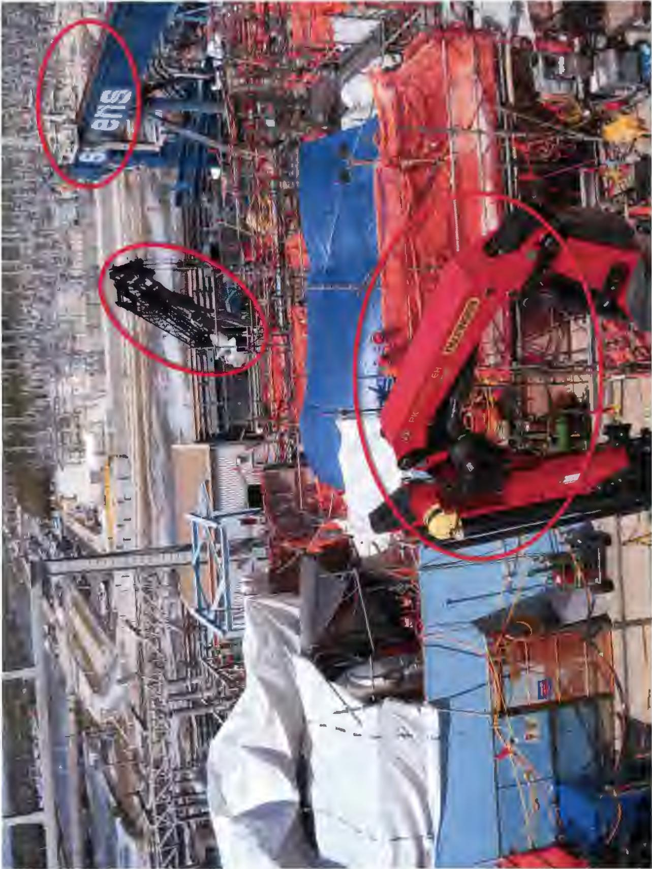
Turkey Point main turbine deck with major components removed on either side of the blue tarp covering the lower casing of the main turbine. The red circles highlight some of the many temporary cranes on site needed to support the work.
