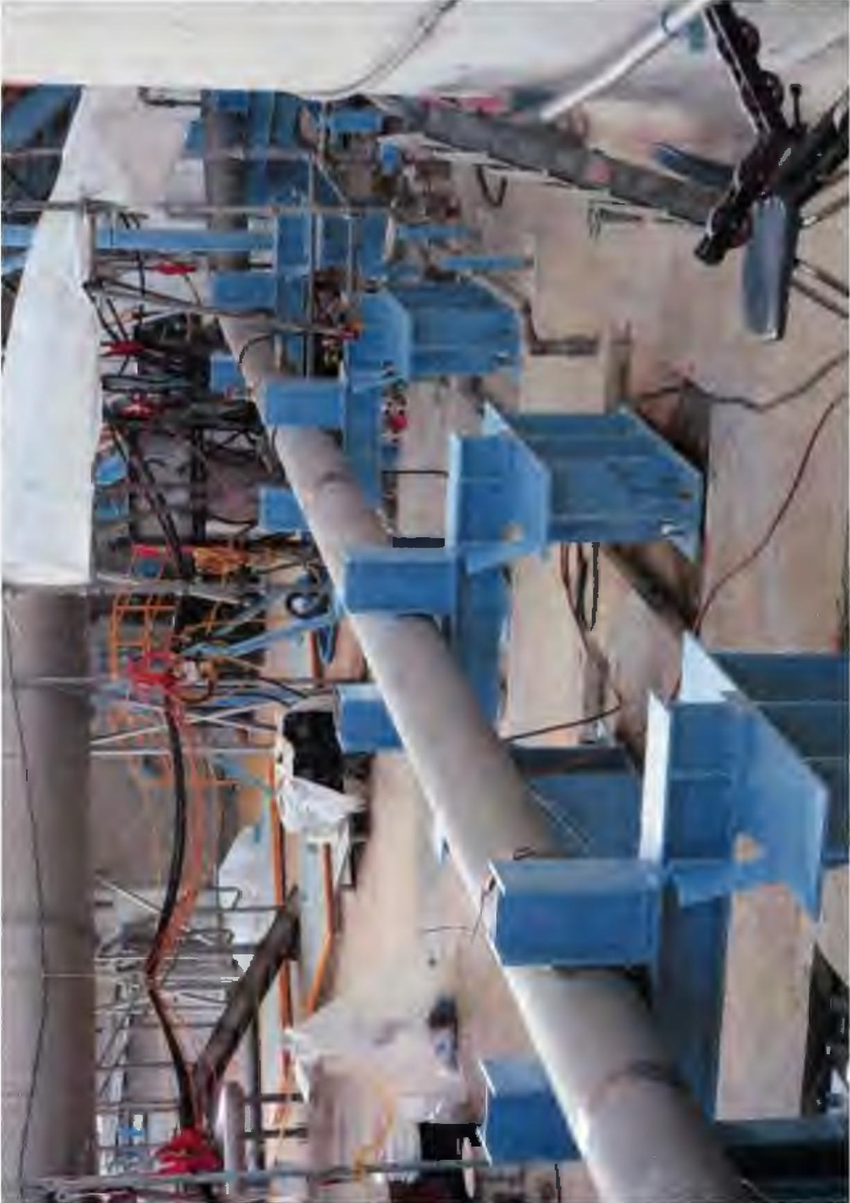
Turkey Point heavy walled ventilation pipe with the many large custom made supports built to design specifications that satisfy regulatory requirements for the CREVS/CREFS systems.
