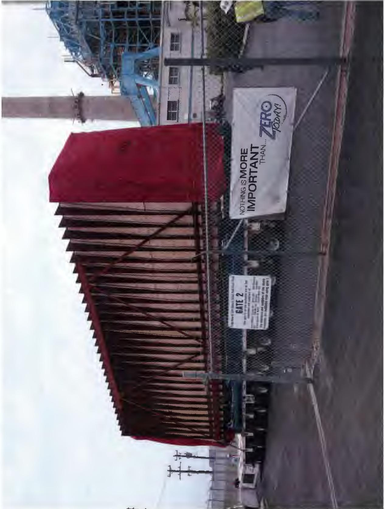
Turkey Point new condenser tube bundle replacement being transported for installation.
