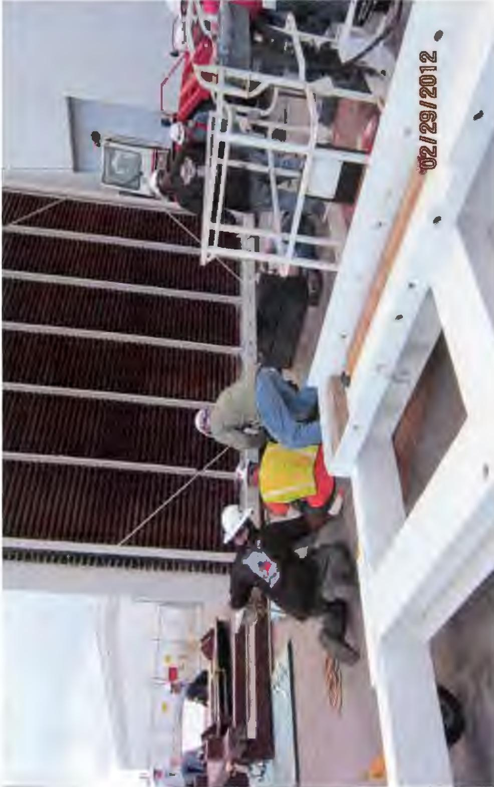
Workers using the new Normal Containment Cooler equipment are practicing installing a cooler outside of the Primary Containment in a clean non-radiological area to reduce assembly time in the Primary Containment radiological control area.
