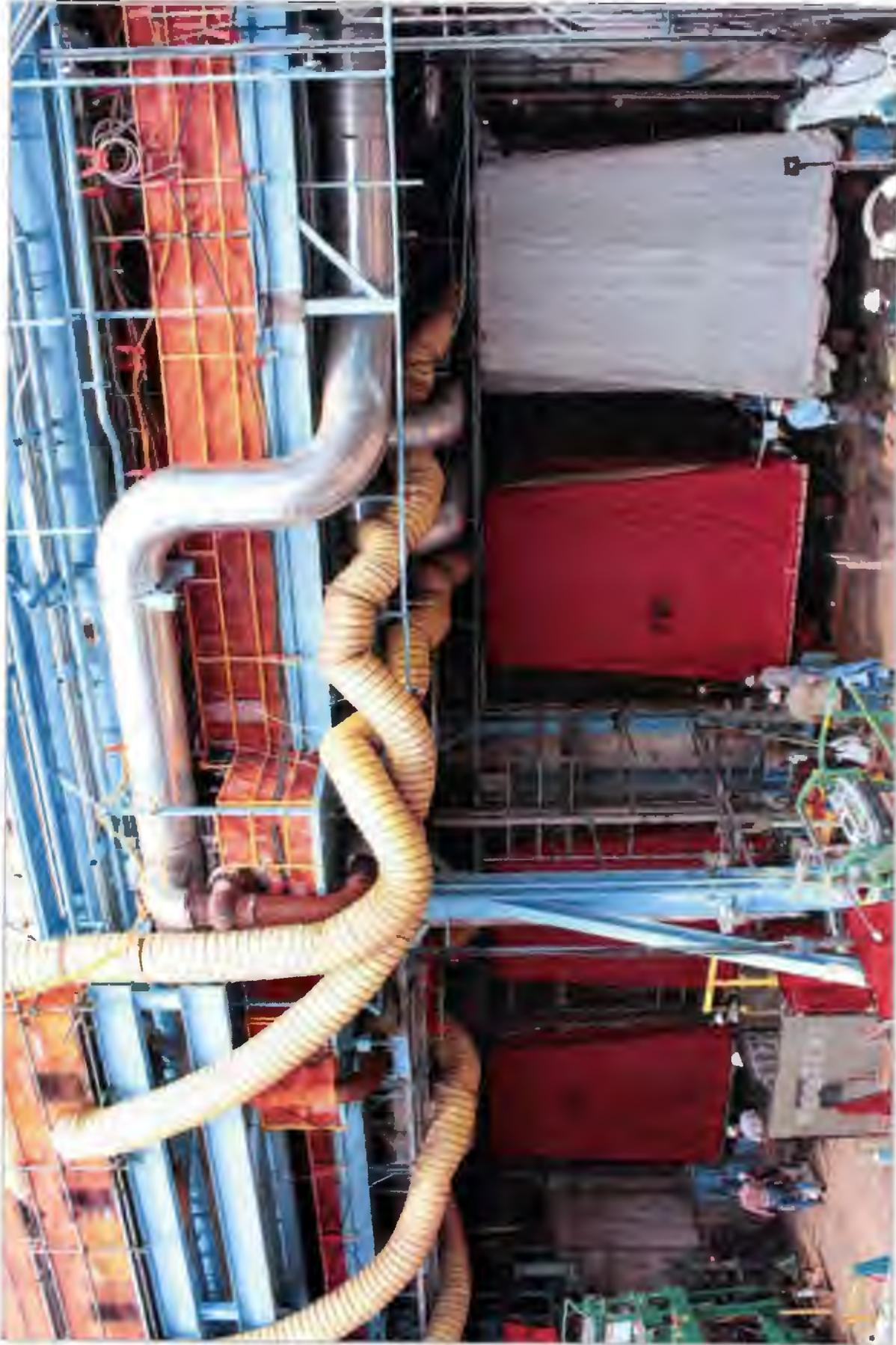
Turkey Point main condenser showing the four condenser sections with the new condenser tube bundles installed.
