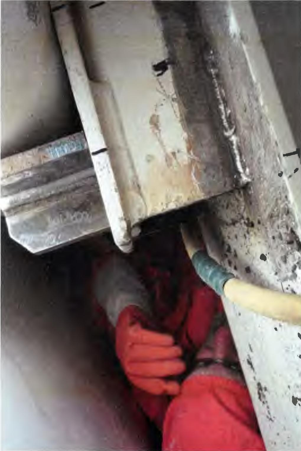
Work inside the containment often place workers in tight, hot spaces. A worker in protective clothing is preparing to weld a support in very close quarters for the Normal Containment Cooler replacement.
