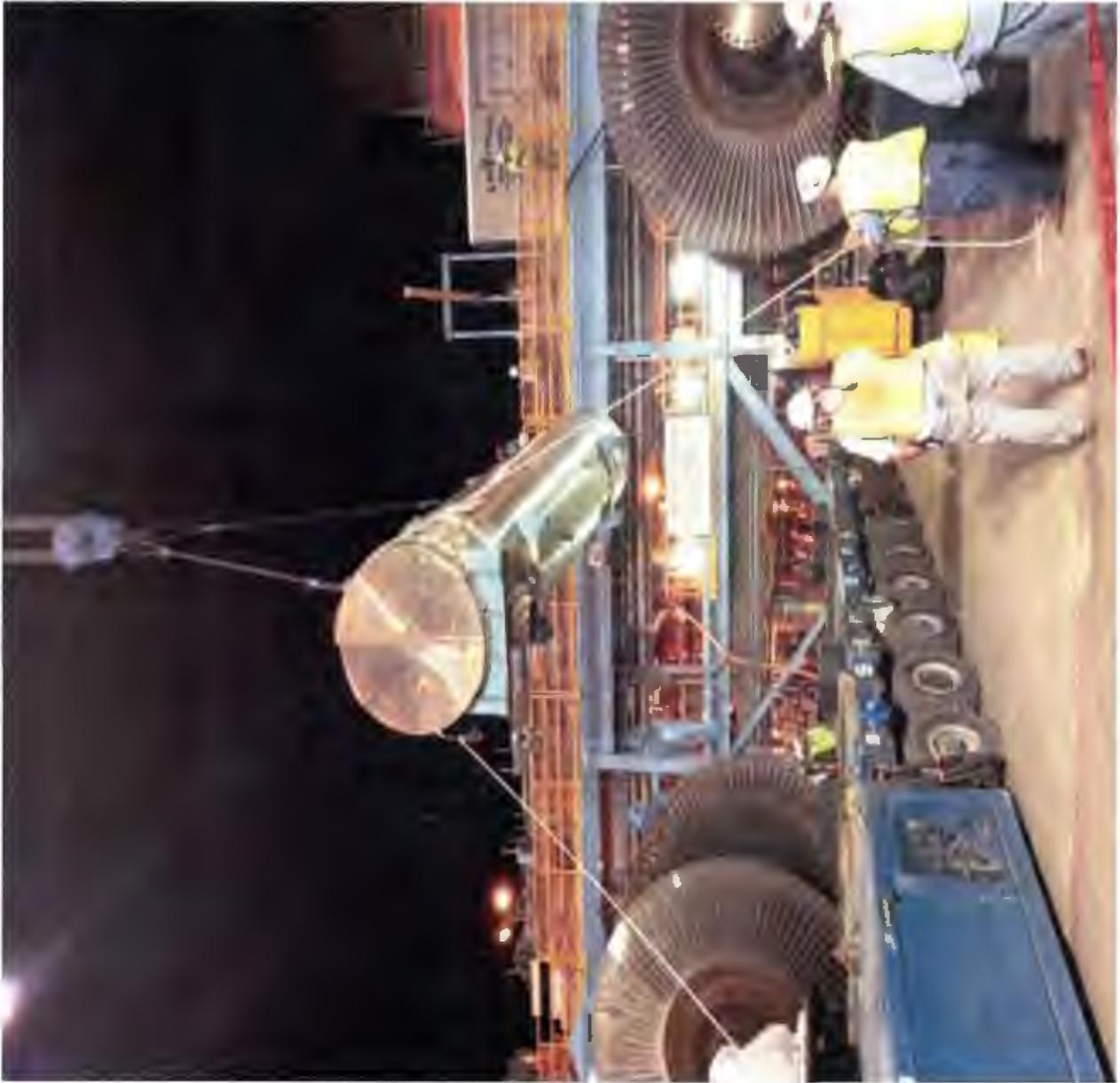
One of four feedwater heaters per unit is being removed from the blue heavy hauler and being staged for lifting onto the turbine deck.
