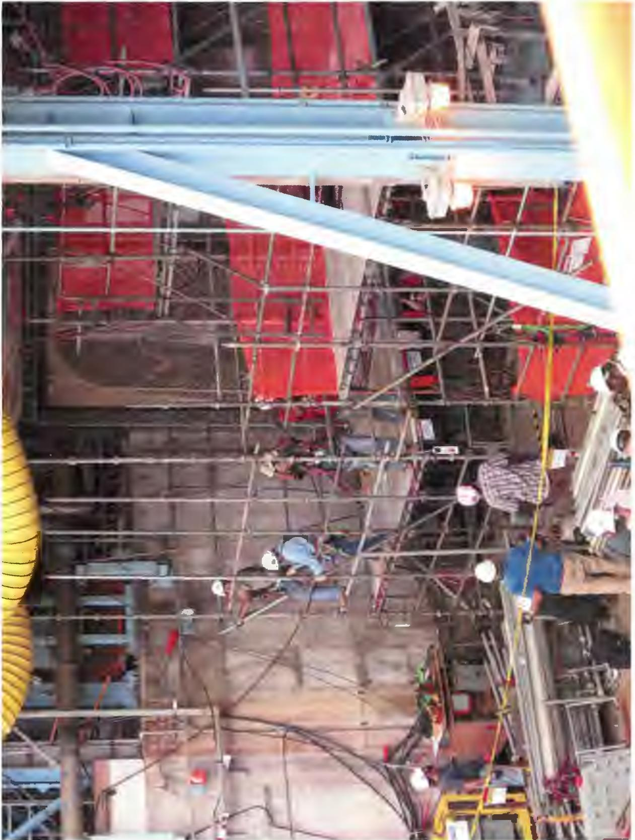
Turkey Point main condenser scaffolding erection to support condenser tube removal.
