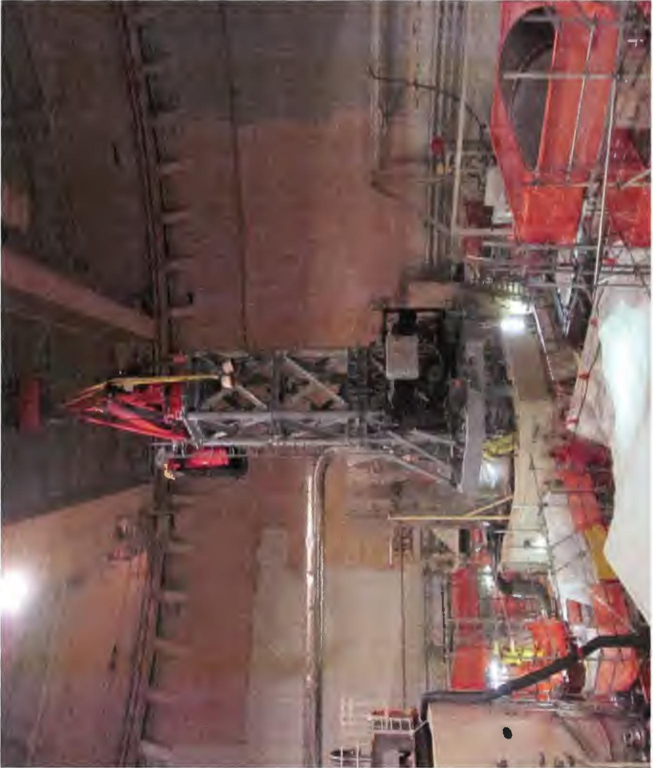
The temporary crane erected in the Primary Containment to support the movement of materials and components.
