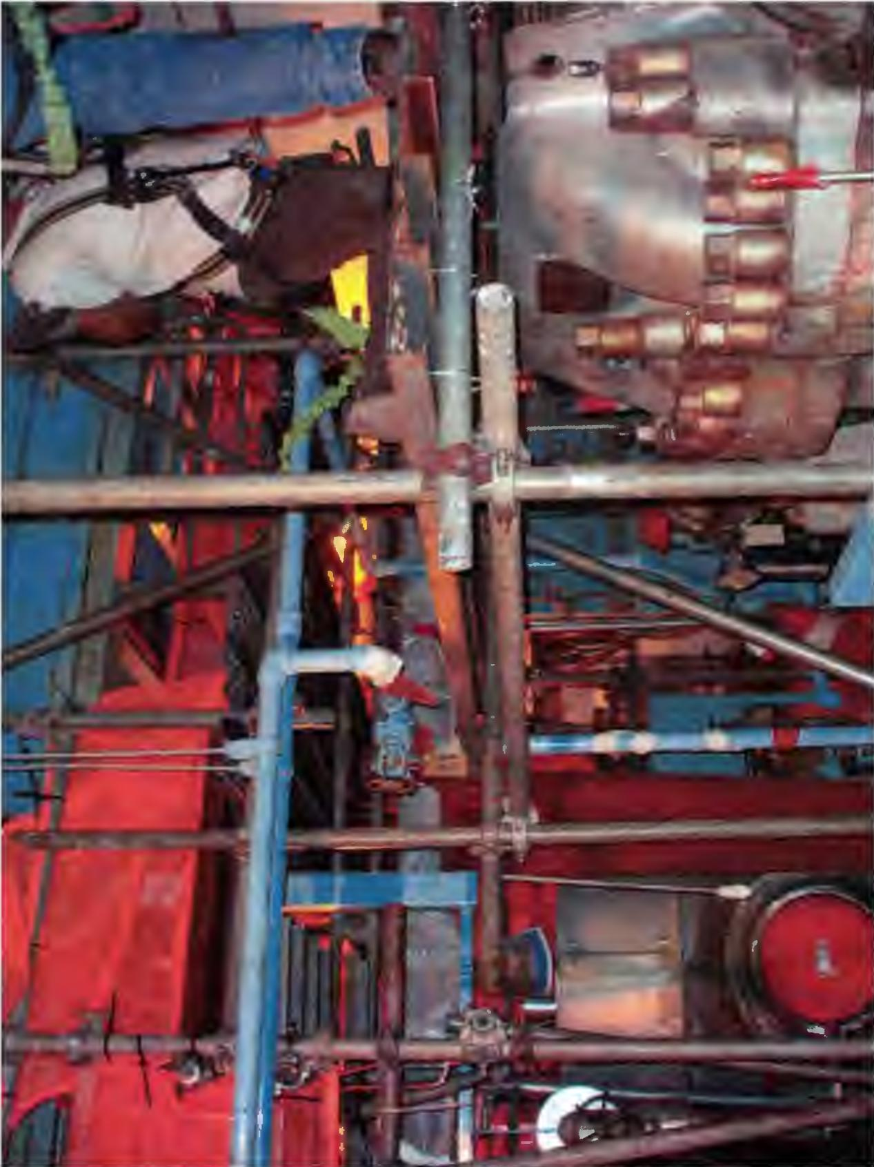
Scaffolding being erected in the congested area around and over one of the Feedwater Pumps
