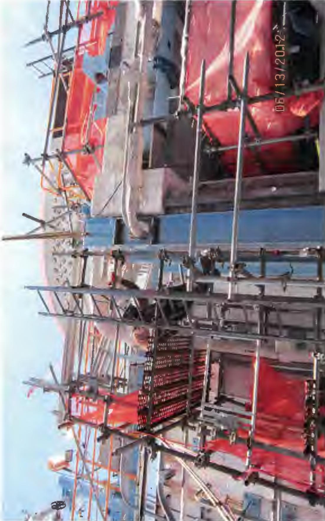
Turkey Point. Scaffolding erected to support the removal of interferences and install the Control Room Emergency Ventilation and Filtration Systems (CREVS/CREFS) with missile protected structures.
