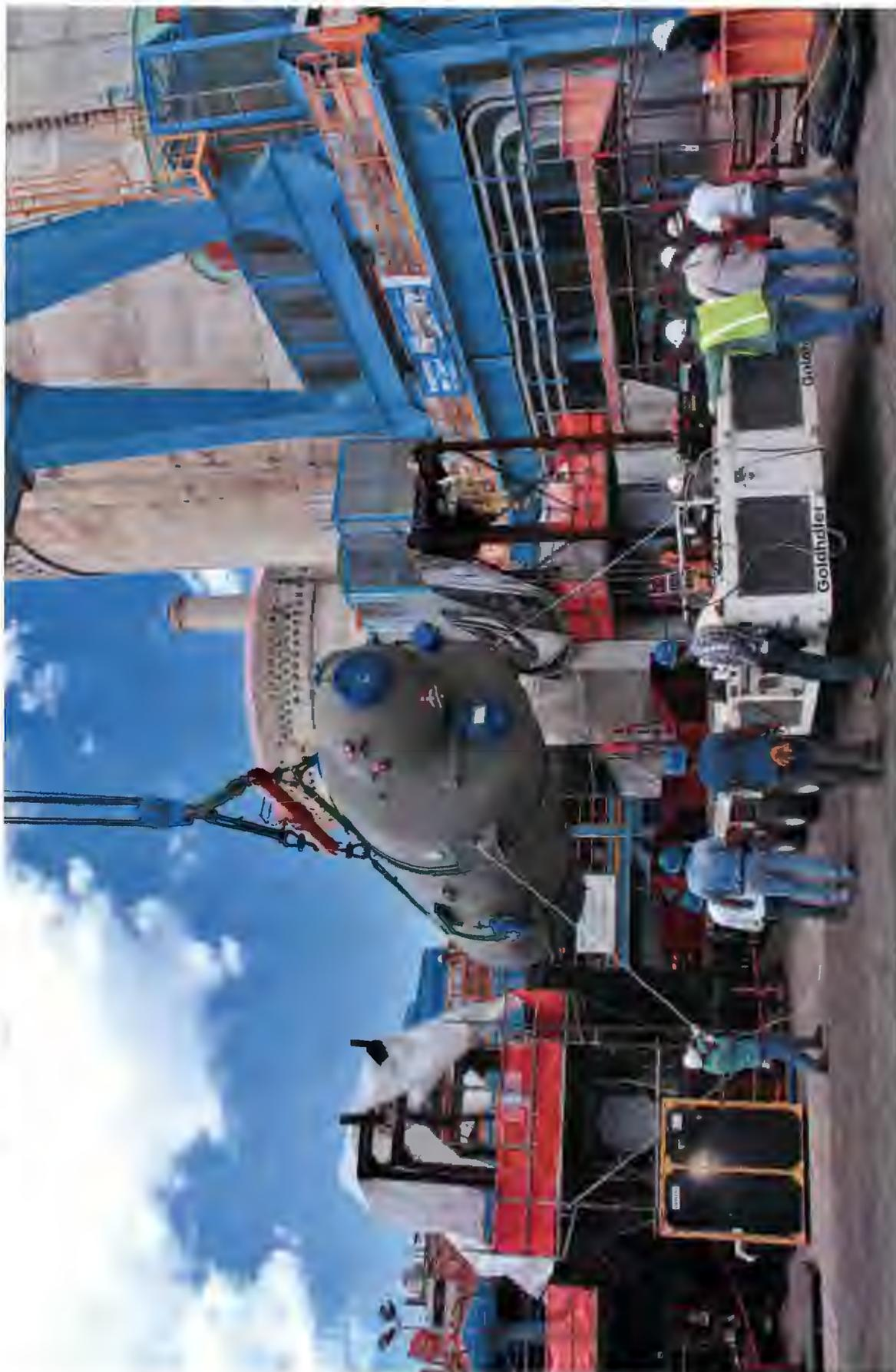
One of the eight Moisture Separators being moved into position on the main turbine deck
