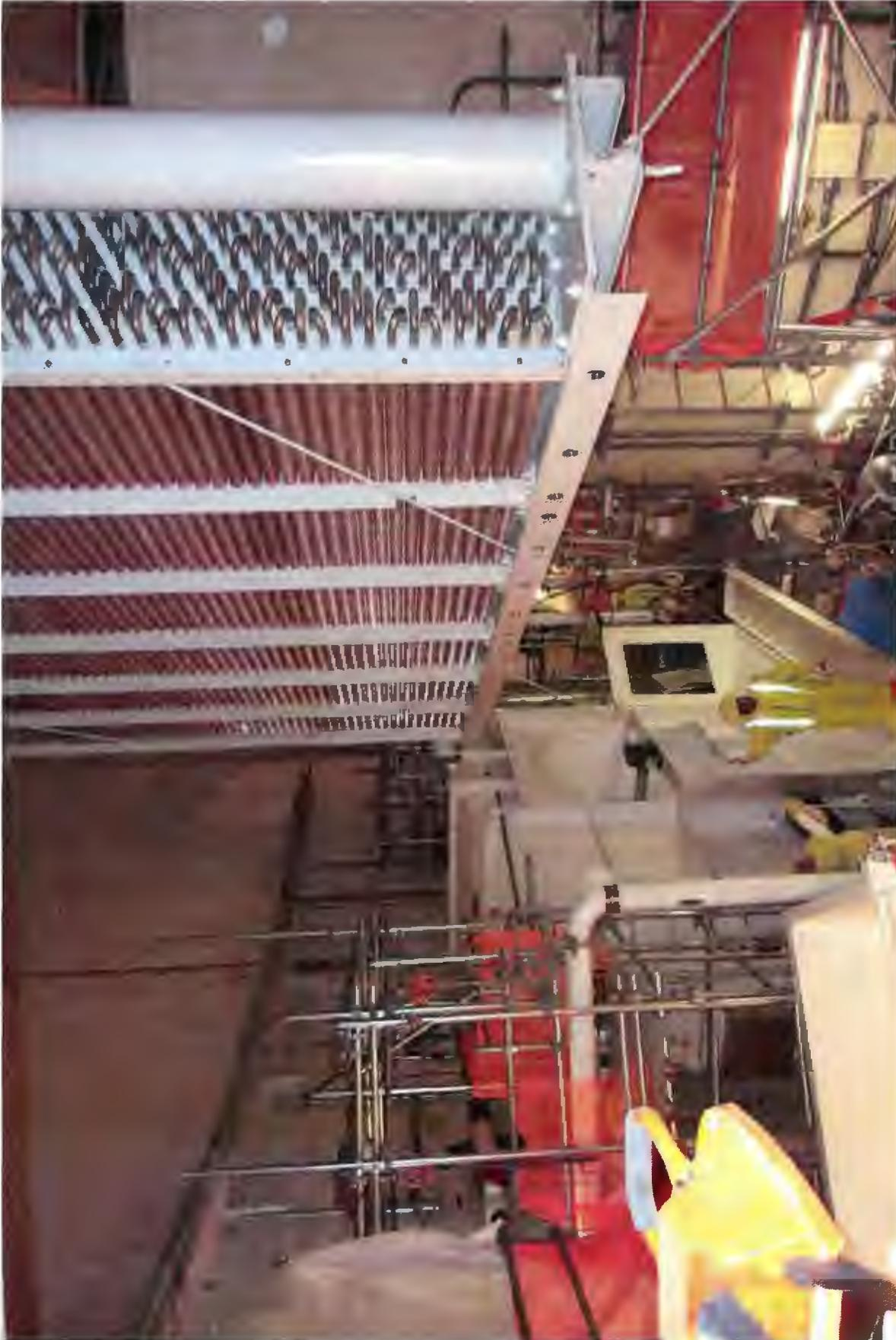
Primary Containment. One of the Normal Containment Coolers being lowered by crane and guided into place by workers using tag lines.
