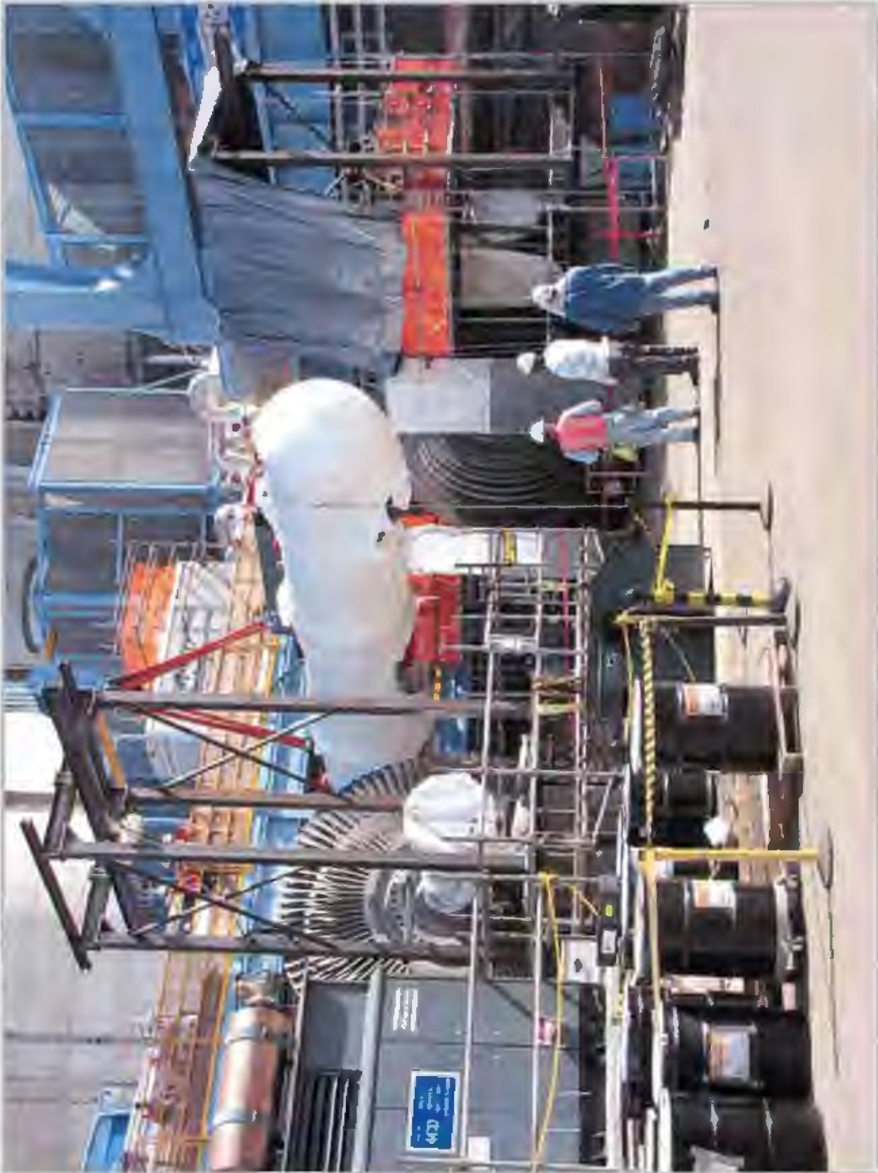
One of four feedwater heaters being lifted by the turbine building crane for placement on the turbine deck.
