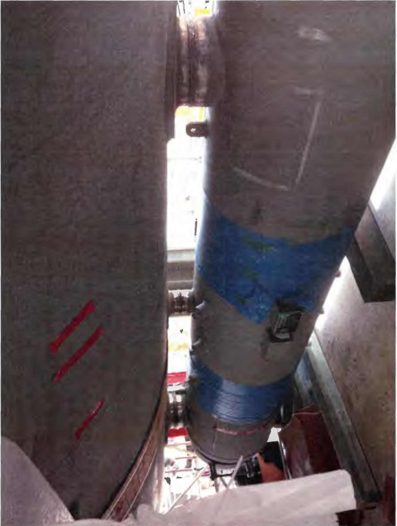
Moisture Separator Drain tank showing welded piping connections to the Moisture Separator Reheater
