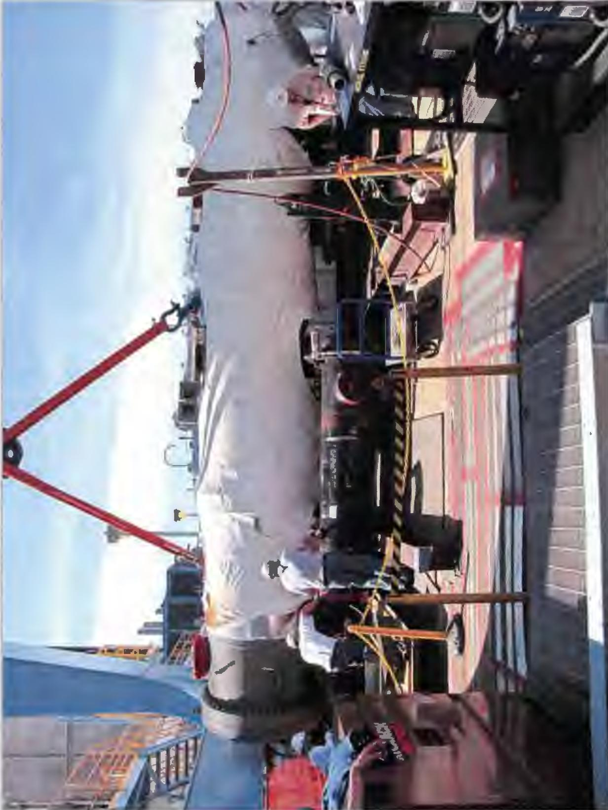
One of the four feedwater heaters being lowered onto beams. Rigging will be attached to the feedwater heater to move it into its location.
