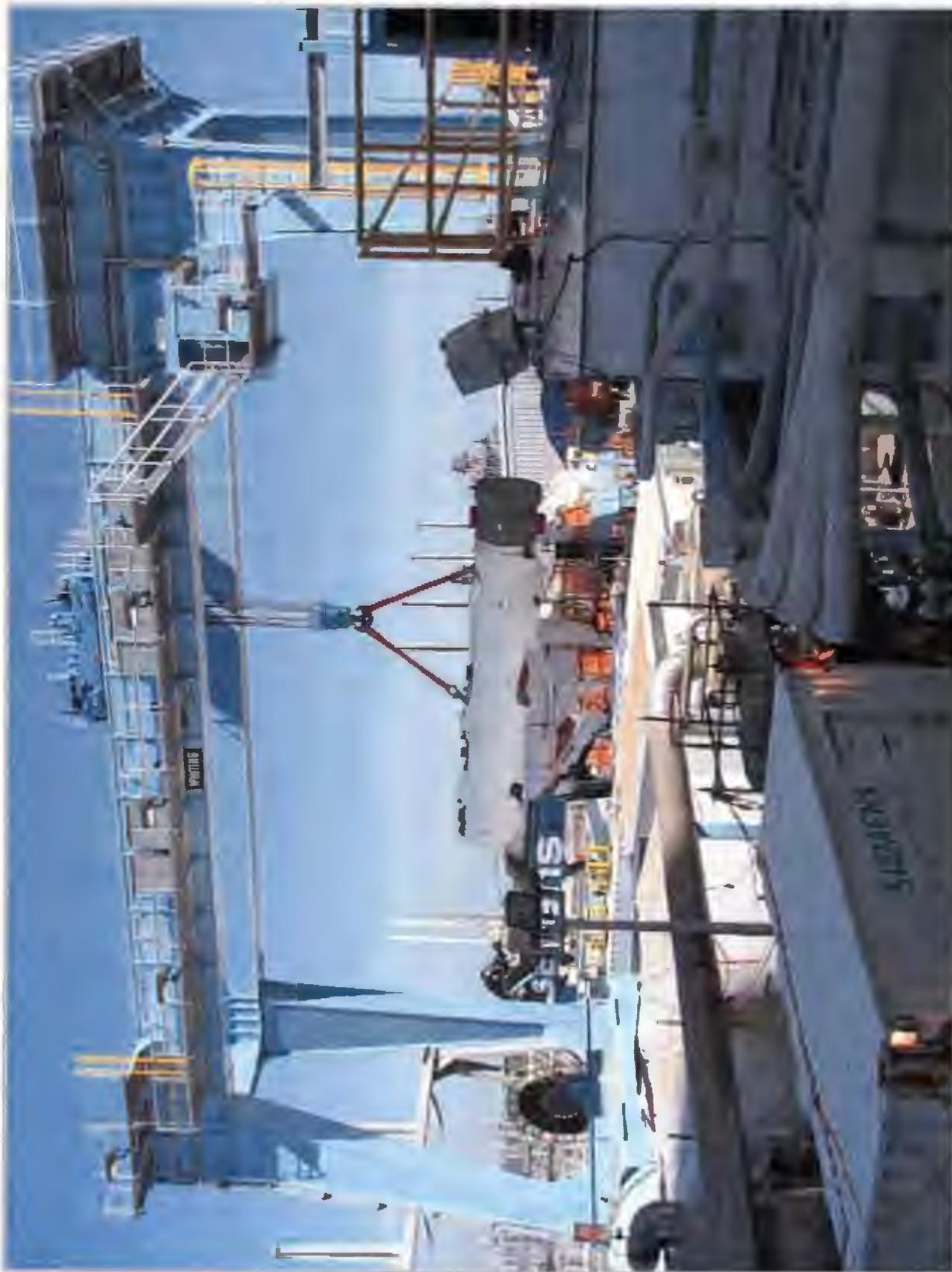
One of four feedwater heaters being moved across the equipment crowded turbine deck for placement on the deck.
