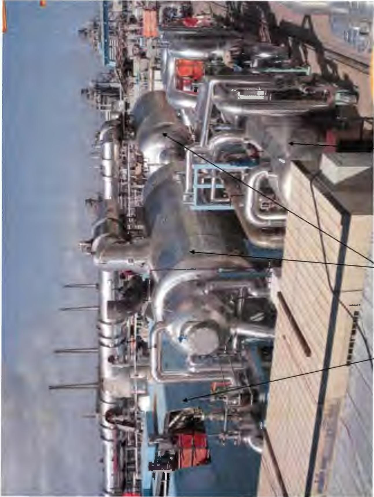
New components installed. High Pressure Turbine, Moisture Separator Reheaters, and High Pressure Feedwater Heater
