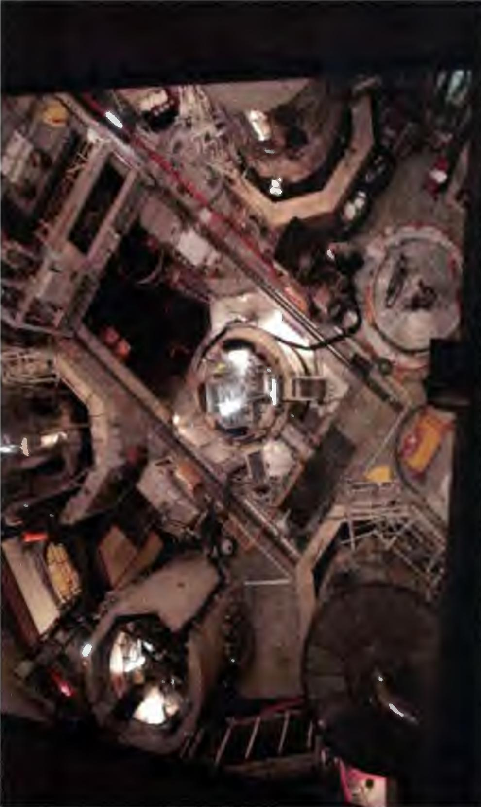
This is the Turkey Point Unit 3 primary containment showing the major components, the Reactor Vessel in the center, the 3 Steam Generators, lower left, upper center and right, and the Pressurizer on the left. A very sturdy platform was installed over the reactor cavity to provide lay down and staging area for the Normal Containment Cooler modification.
