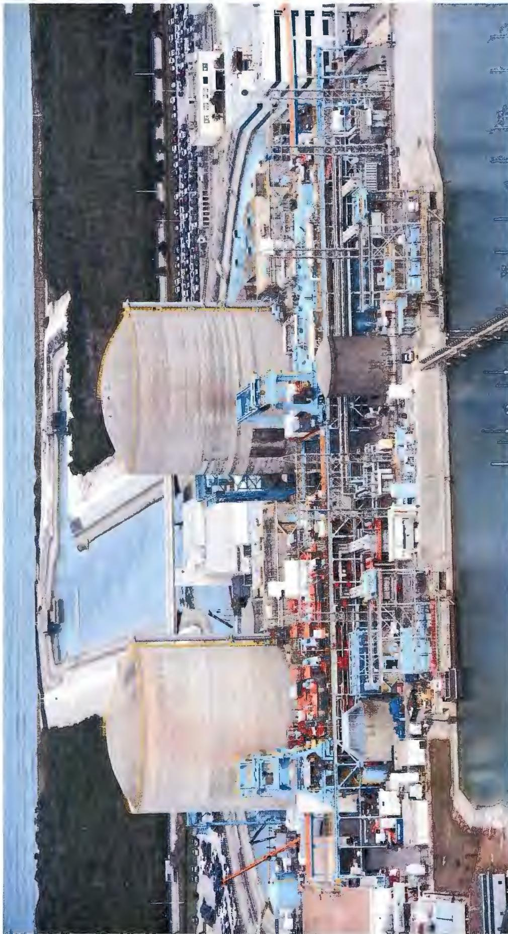
St. Lucie Unit 1 on left shows the early stage of mobilization of safety barriers in advance of demolition, compared to Unit 2 (on right) which is in operation
