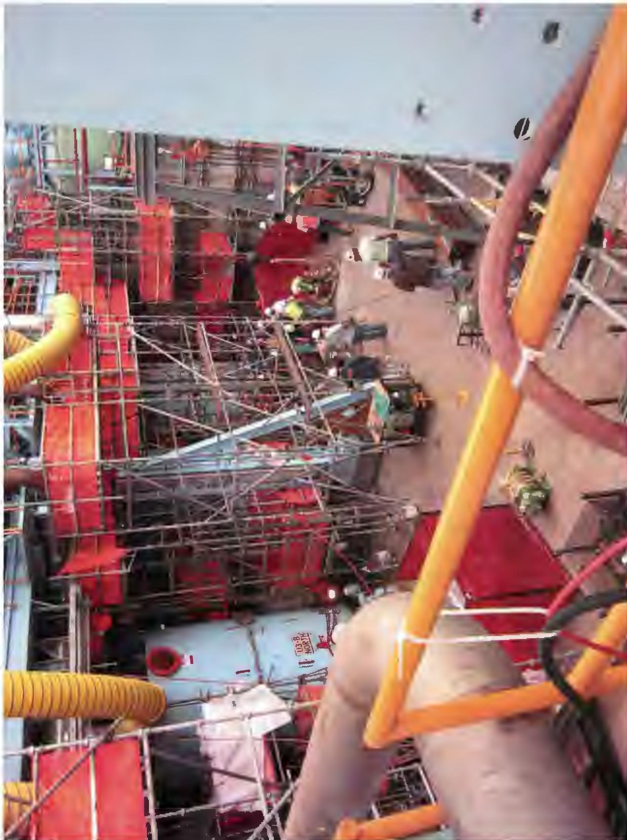
Turkey Point Main Condenser. Scaffolding being erected to support the Main Condenser Replacement modification.
