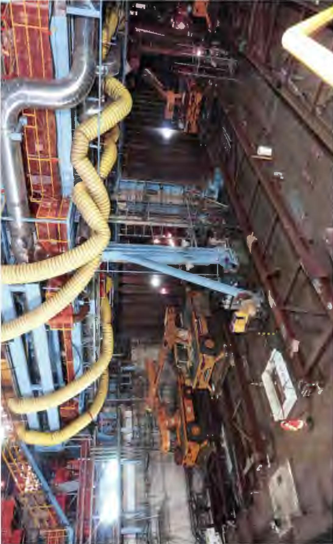
Turkey Point main condenser area with the old condenser demolished and preparations being made to install the new condenser tube bundle.
