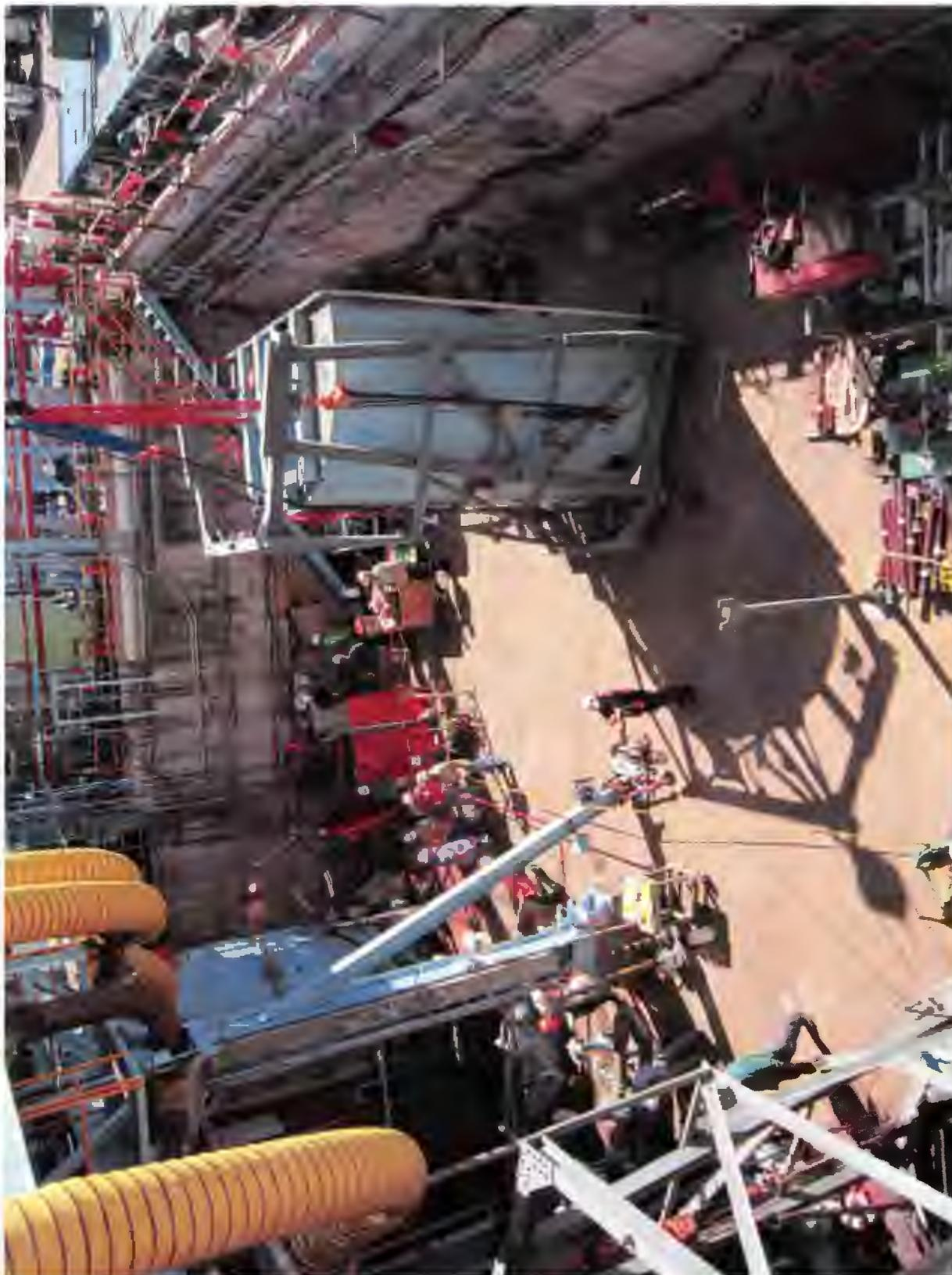
Turkey Point Main Condenser canal cooling water box removal to expose the tens of thousands of condenser tubes for removal.
