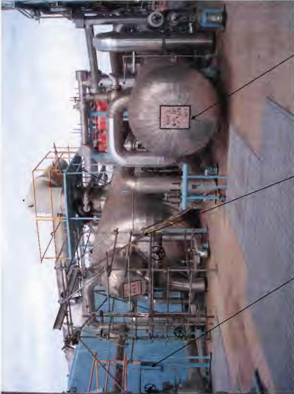
Turkey Point Main Turbine Deck showing the High Pressure Turbine enclosure, 1 of 4 Moisture Separator Reheaters and 1 of 2 of the 6A (B) High Pressure Feedwater Heaters, before EPU. All of these components were demolished and new larger equipment was installed to produce more power.
