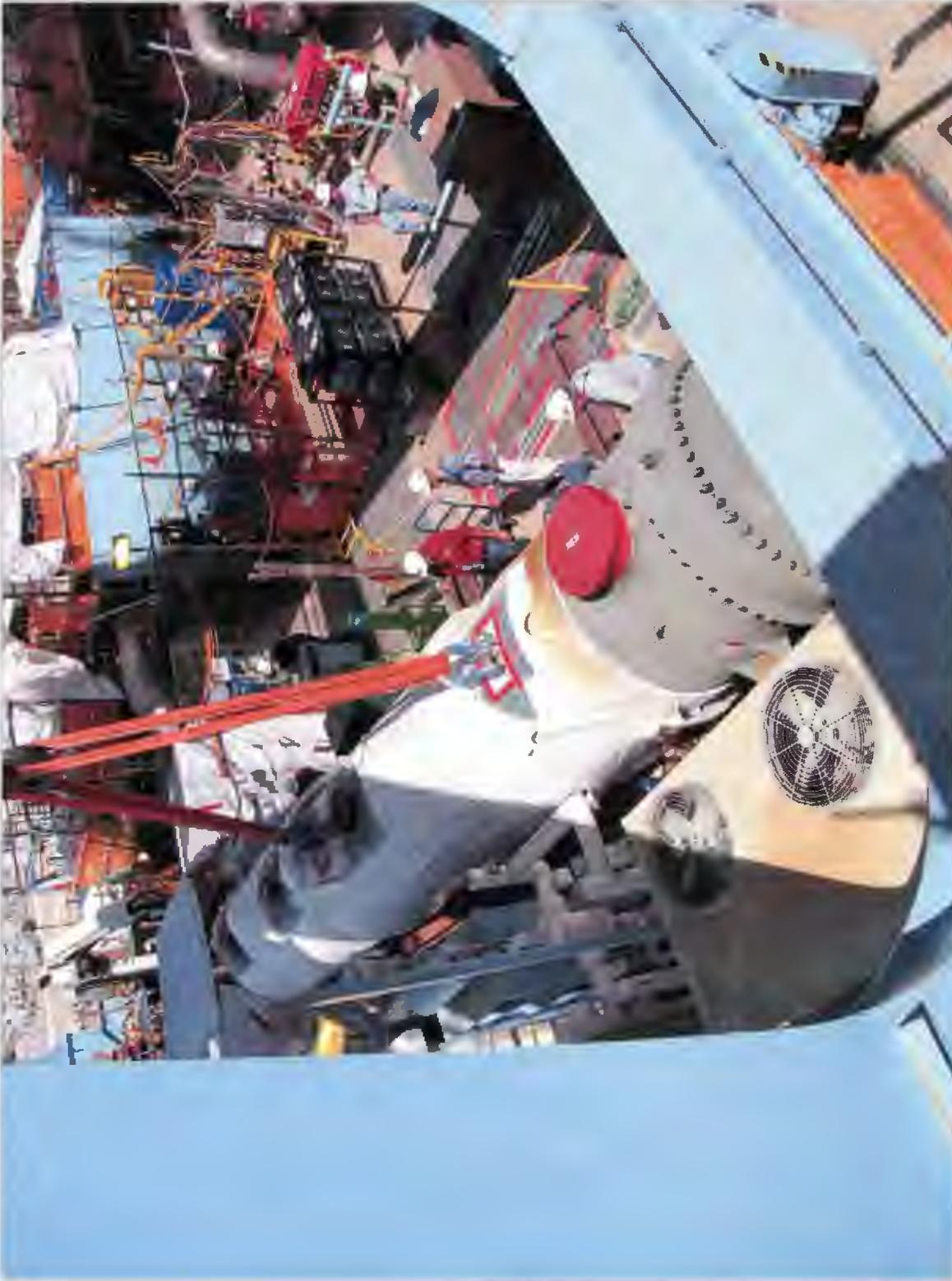
One of four feedwater heaters being lowered into the close-quarters of the turbine deck, where it will then be moved to its location.
