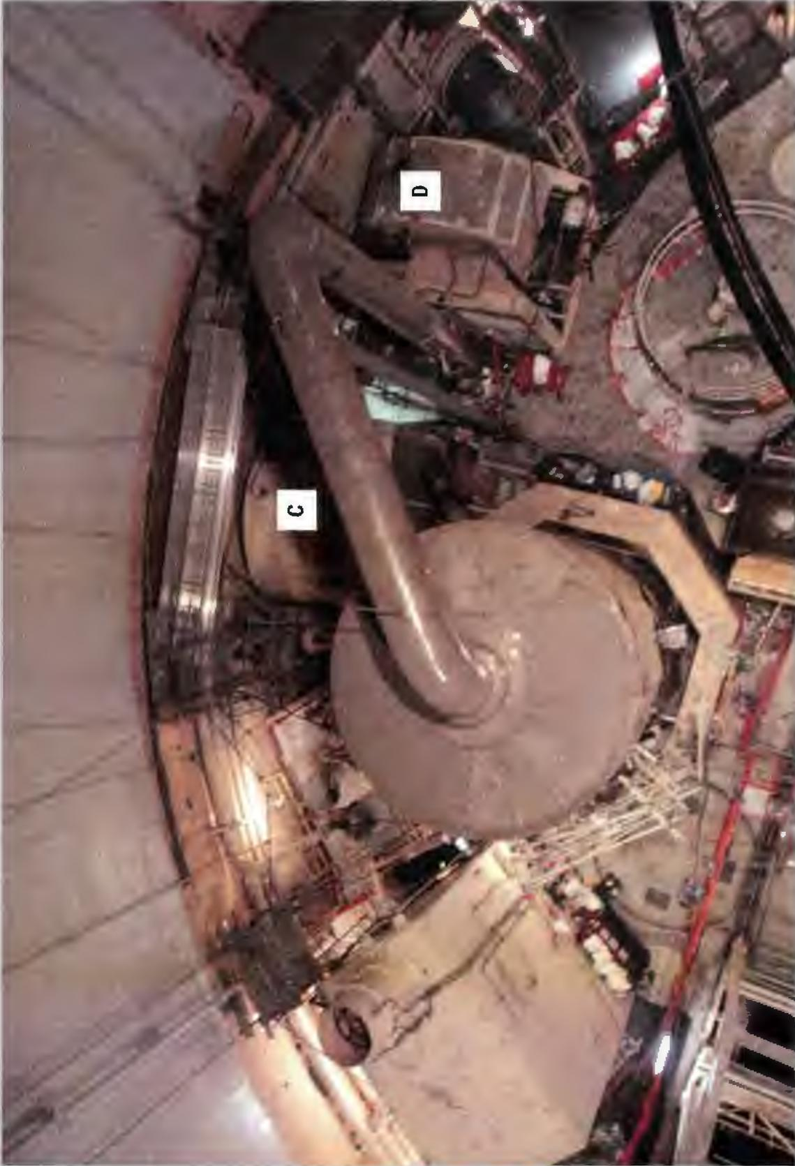
The equipment and components located inside the primary containment generate a tremendous amount of additional heat. For that reason all four normal containment coolers (two pictured above) were replaced with newer models in both units. This will increase the cooling capacity inside the reactor buildings.
