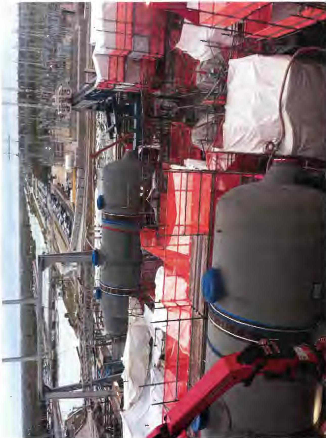
Two of the eight new Moisture Separators in their location on the Main Turbine Deck
