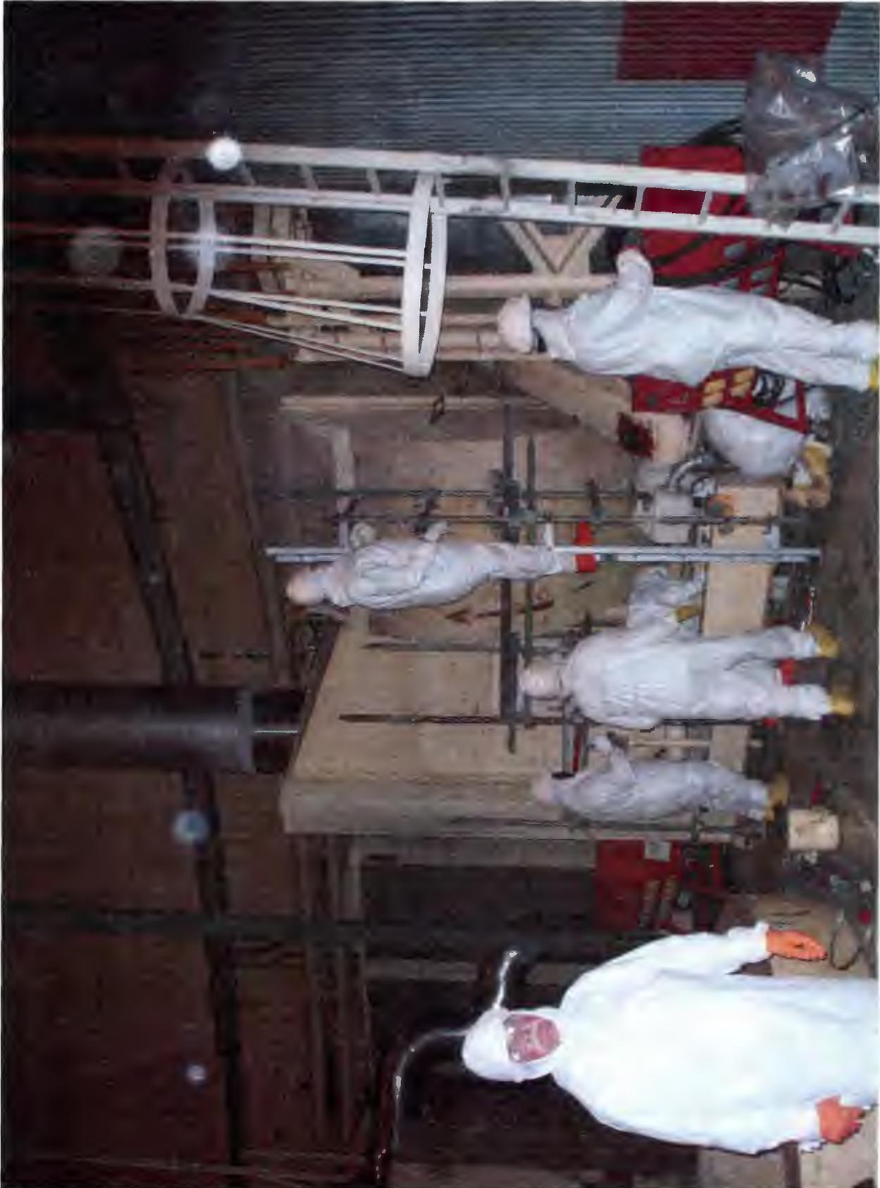
Turkey Point Normal Containment Coolers demolition. Workers are in Radioactive Contamination Protective Clothing erecting needed scaffolding.
