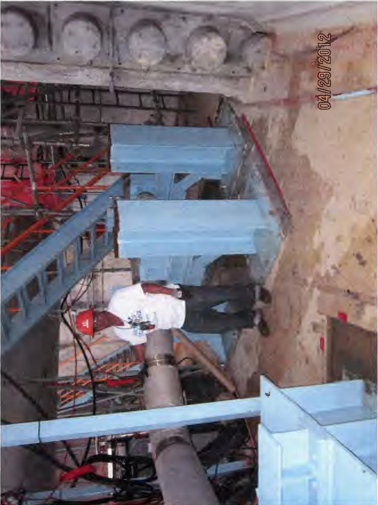
Turkey Point heavy walled emergency ventilation pipe with one of its very large structural supports.
