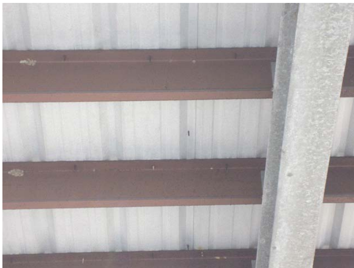
View of structure
