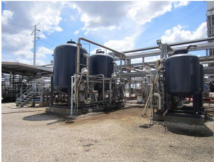
General view of tanks in section
