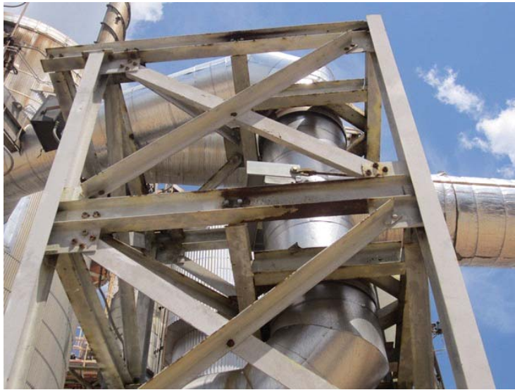
View of structure
