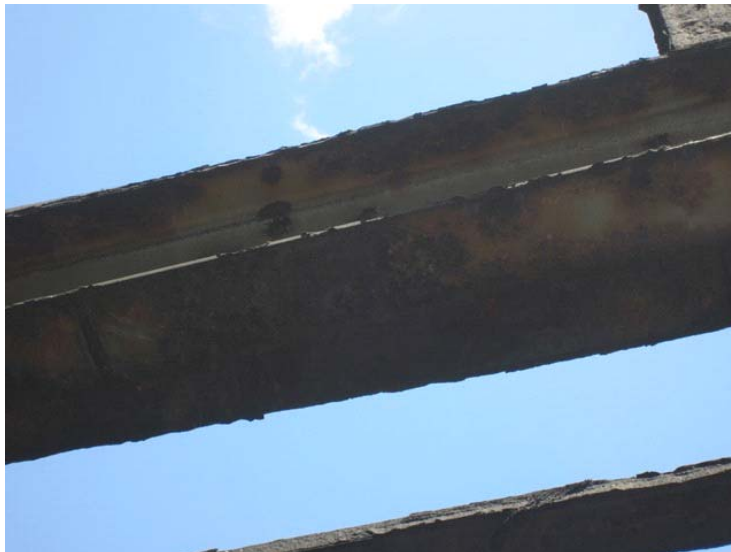
Severe corrosion
