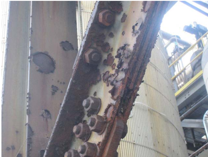
Heavy corrosion
