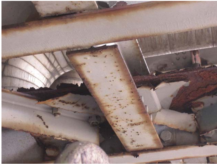
Heavy corrosion
