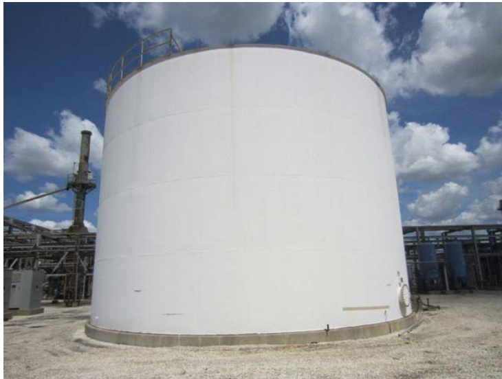
General view of tank in section
