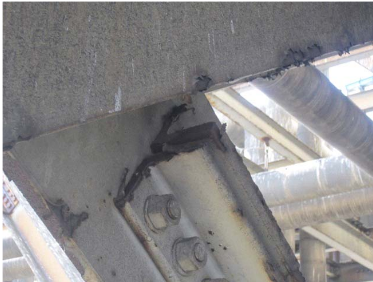
Undercutting visible
