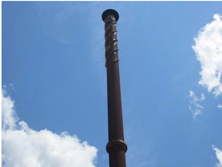
General view of stack
