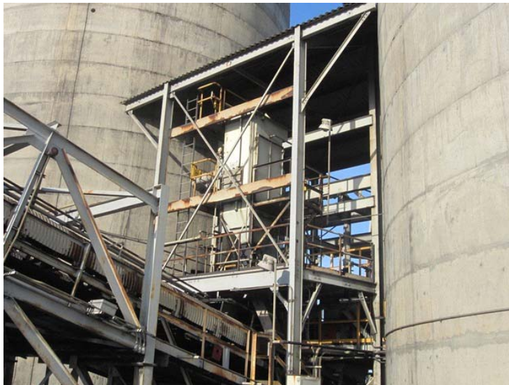
General view of structure
