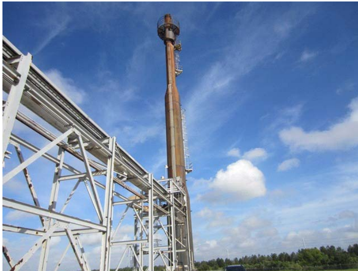
General view of stack
