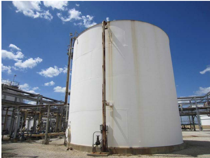
General view of tank
