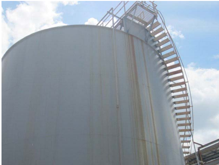
General view of Tank
