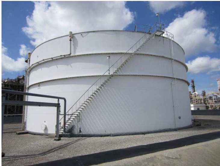
General view of tank
