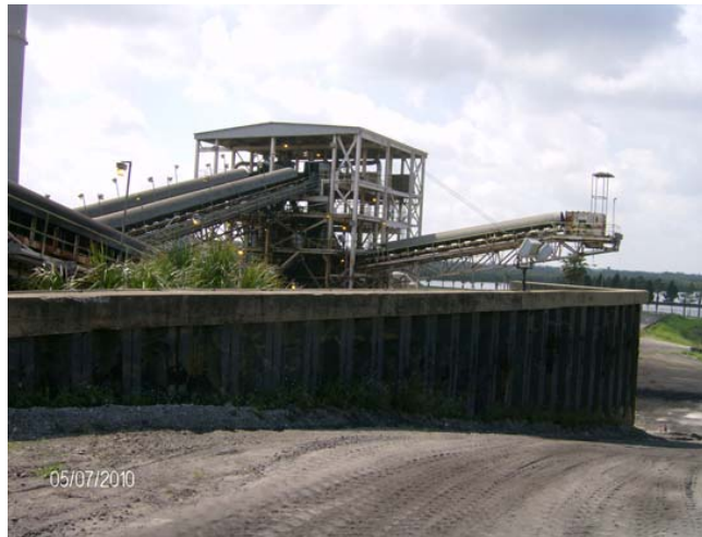
Transfer Tower T7
