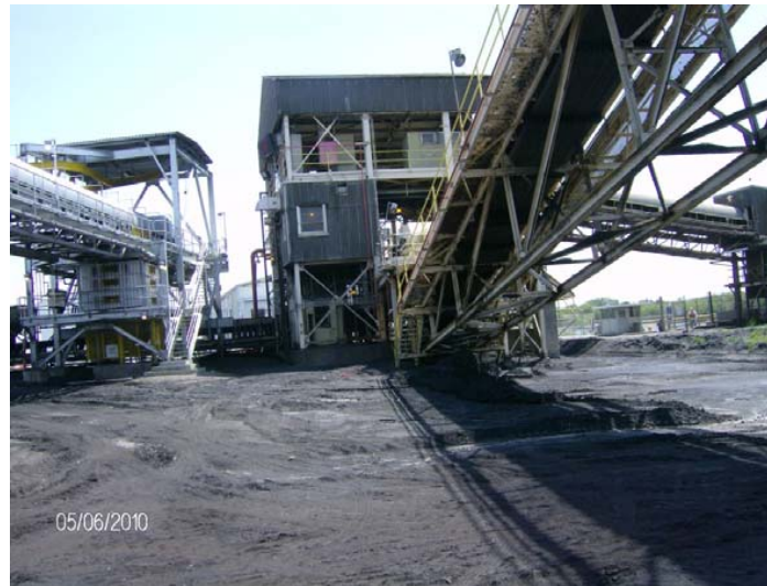
T2 Transfer Tower
