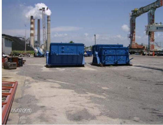
Coal Crushers ready for installation
