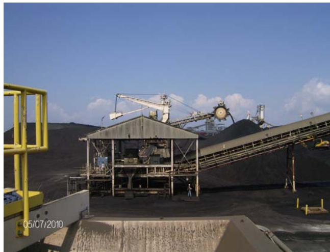
T3 Transfer Tower
