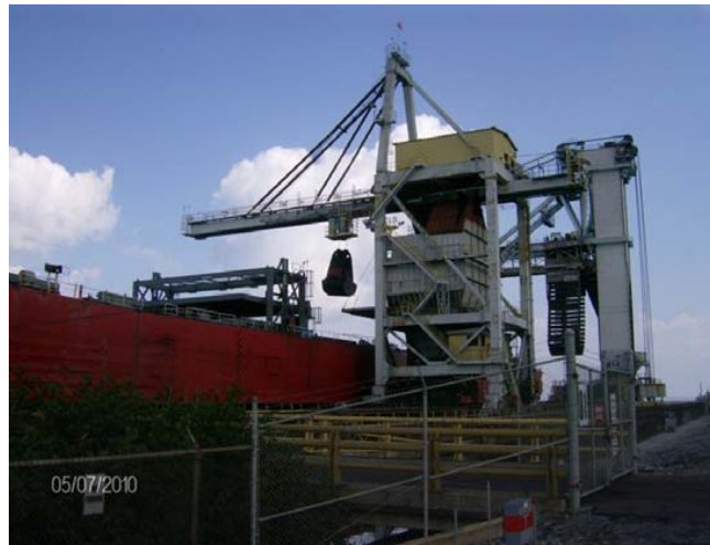
PECO Unloader (foreground)
