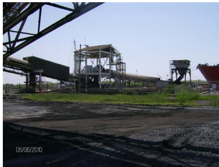
T1 Transfer Tower
