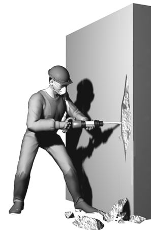
Fig. 2—Bulk concrete removal.
