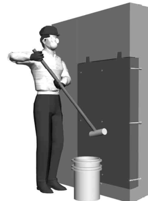
Fig. 4—Material placement: vertical application.
