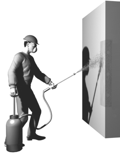
Fig. 9—Spray application of curing compound.
