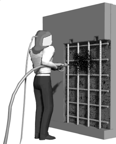
Cleaning of reinforcing steel and concrete with abrasive blast.
