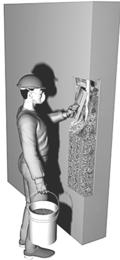
Fig. 8—Hand application of repair material.
