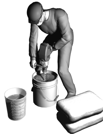
Fig. 7—Typical equipment to mix materials.
