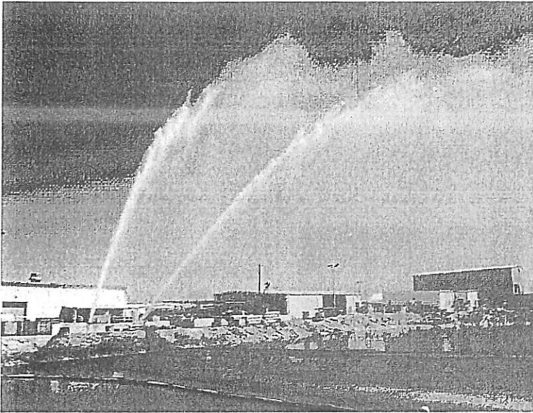
High-pressure water cannons are tested as part of plant emergency readiness.
