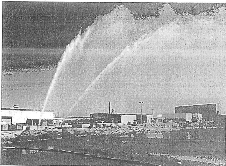
High-pressure water cannons are tested as part of plant emergency readiness.
