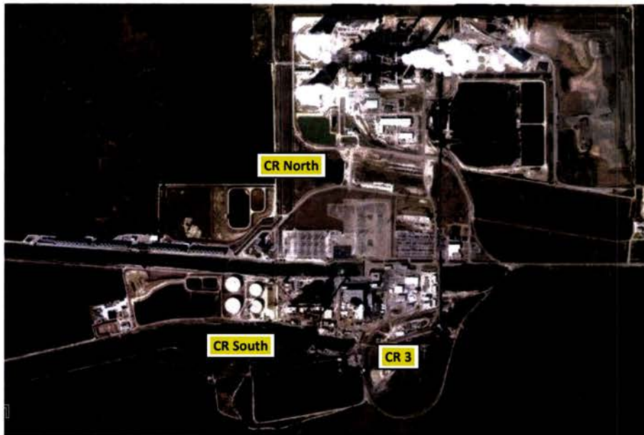
Figure 1-1 Crystal River Energy Complex
