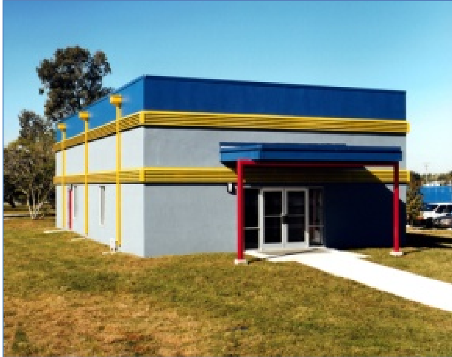
Figure 1. The Building Science Lab is a 2000 ft 2 , highly instrumented lab building located on the FSEC campus.
