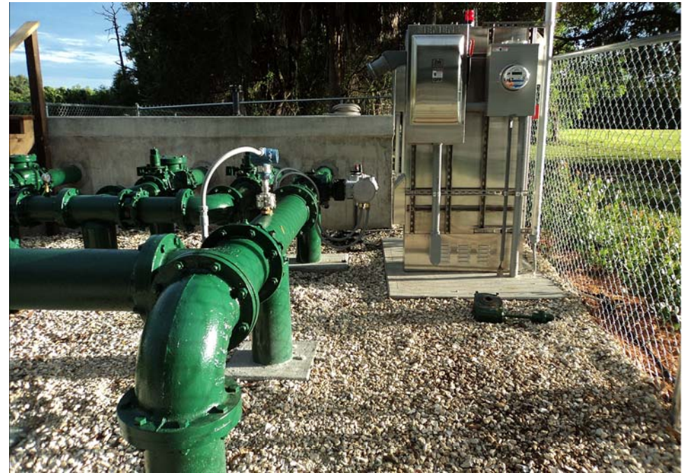
INFLUENT LINE AND MOTORIZED CONTROL VALVE
