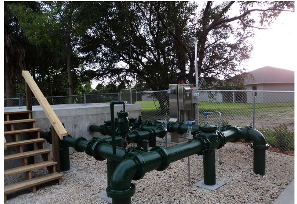
INFLUENT LINE AND MOTORIZED CONTROL VALVE
