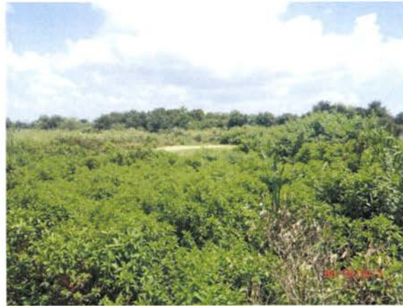
4 Severely overgrown percolation pond
