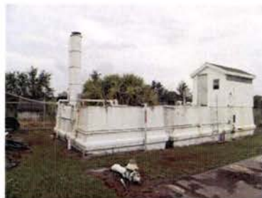
Tree between ground storage tanks and the pipe to the old hydro tank
