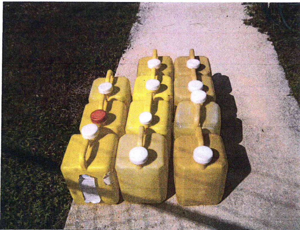
On-Site Chlorine Supply
