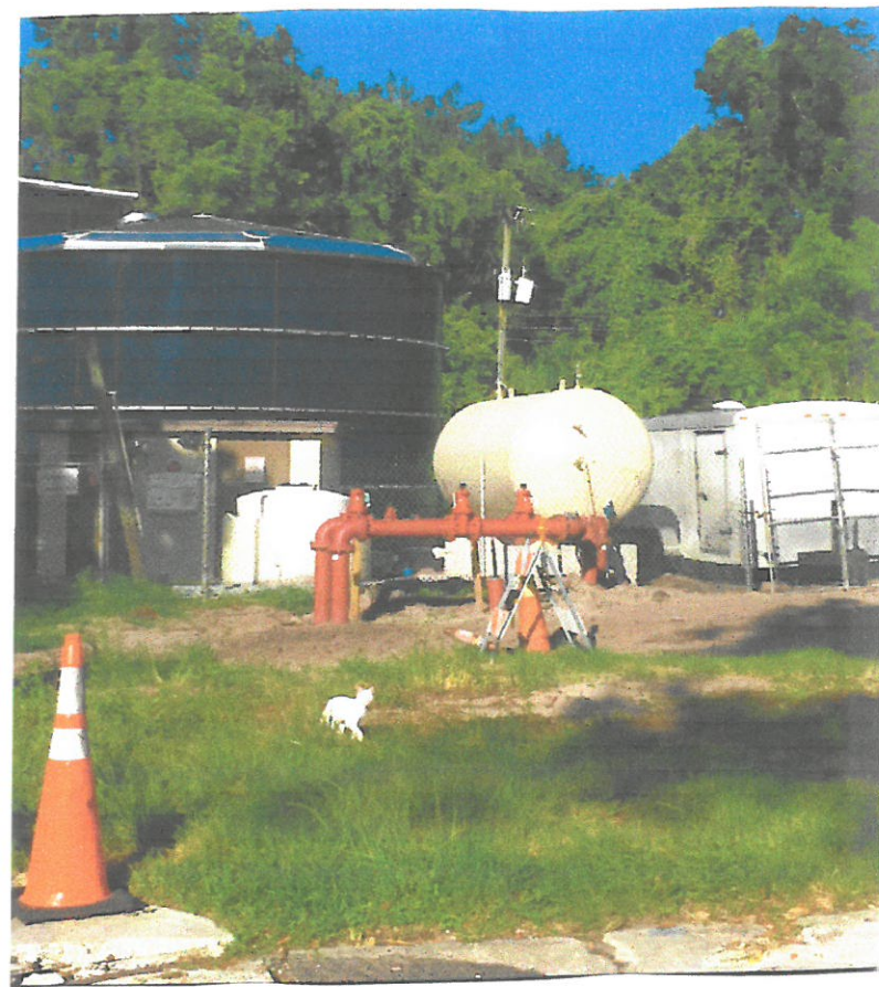
Work on plant by house on Temple Dr.
