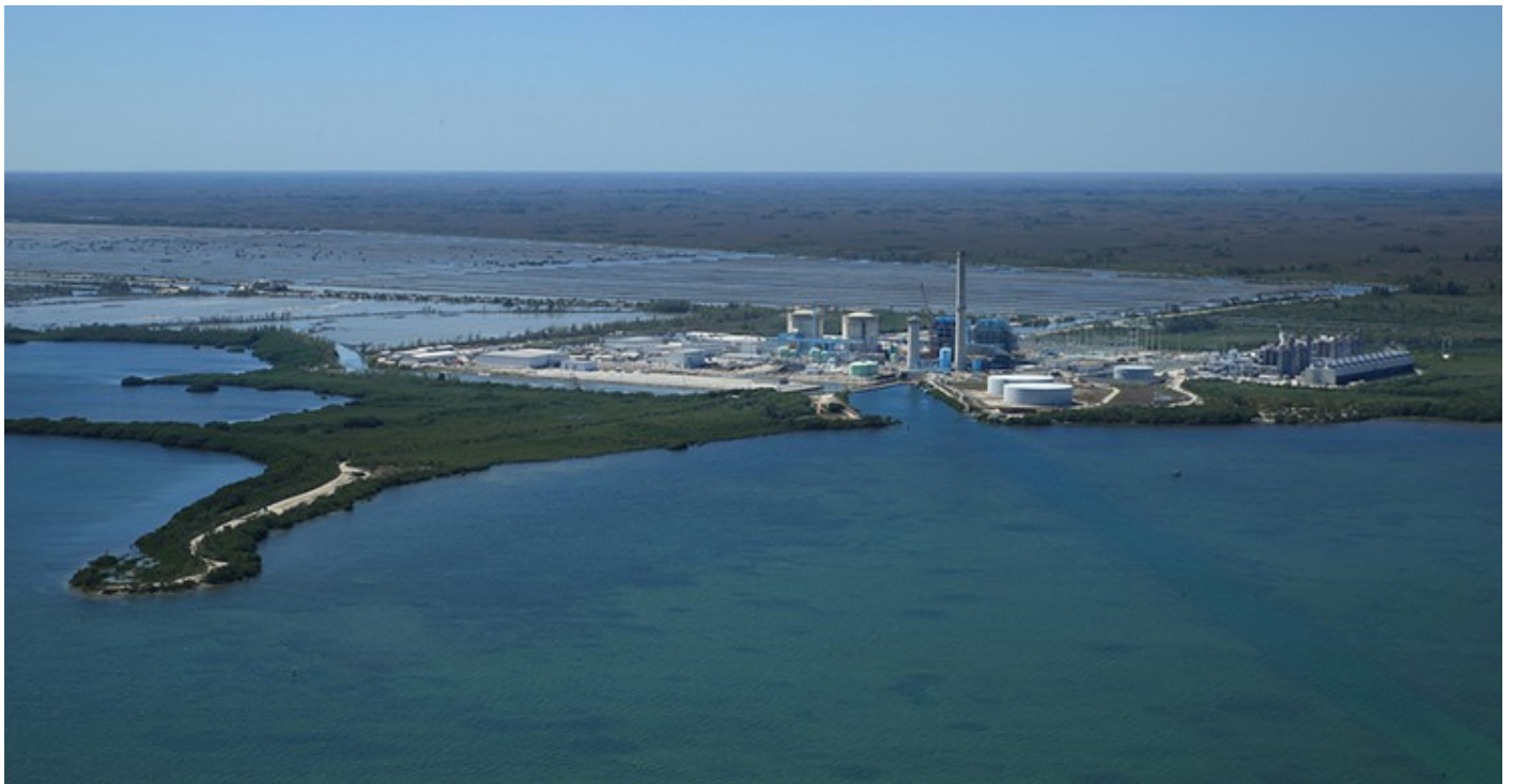
The reactors at Turkey Point are two squat, round structures at the center of the photo.
