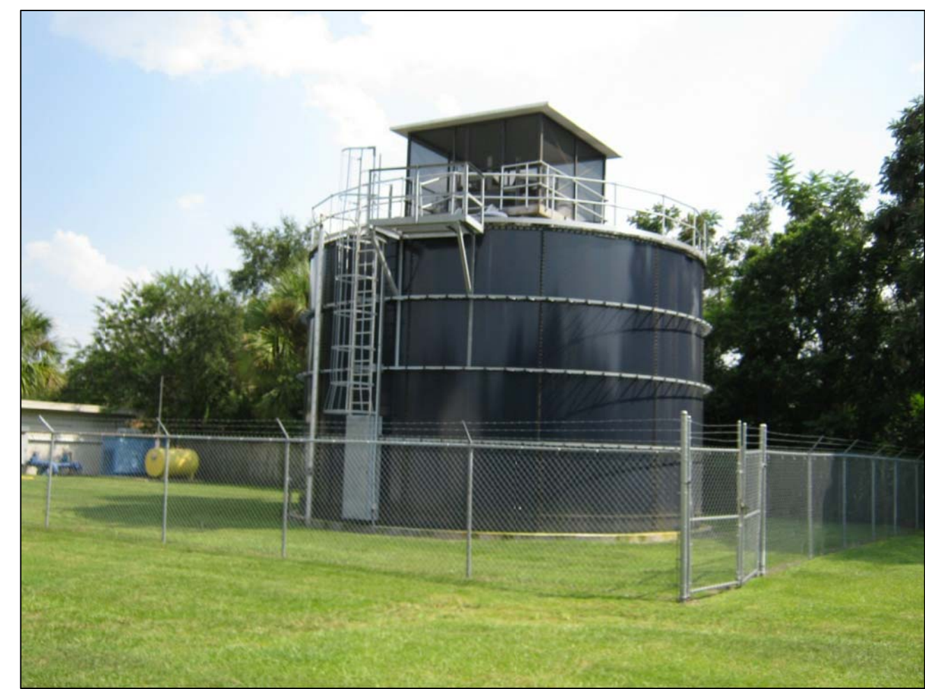
4 WEATHERSFIELD WATER TREATMENT PLANT
