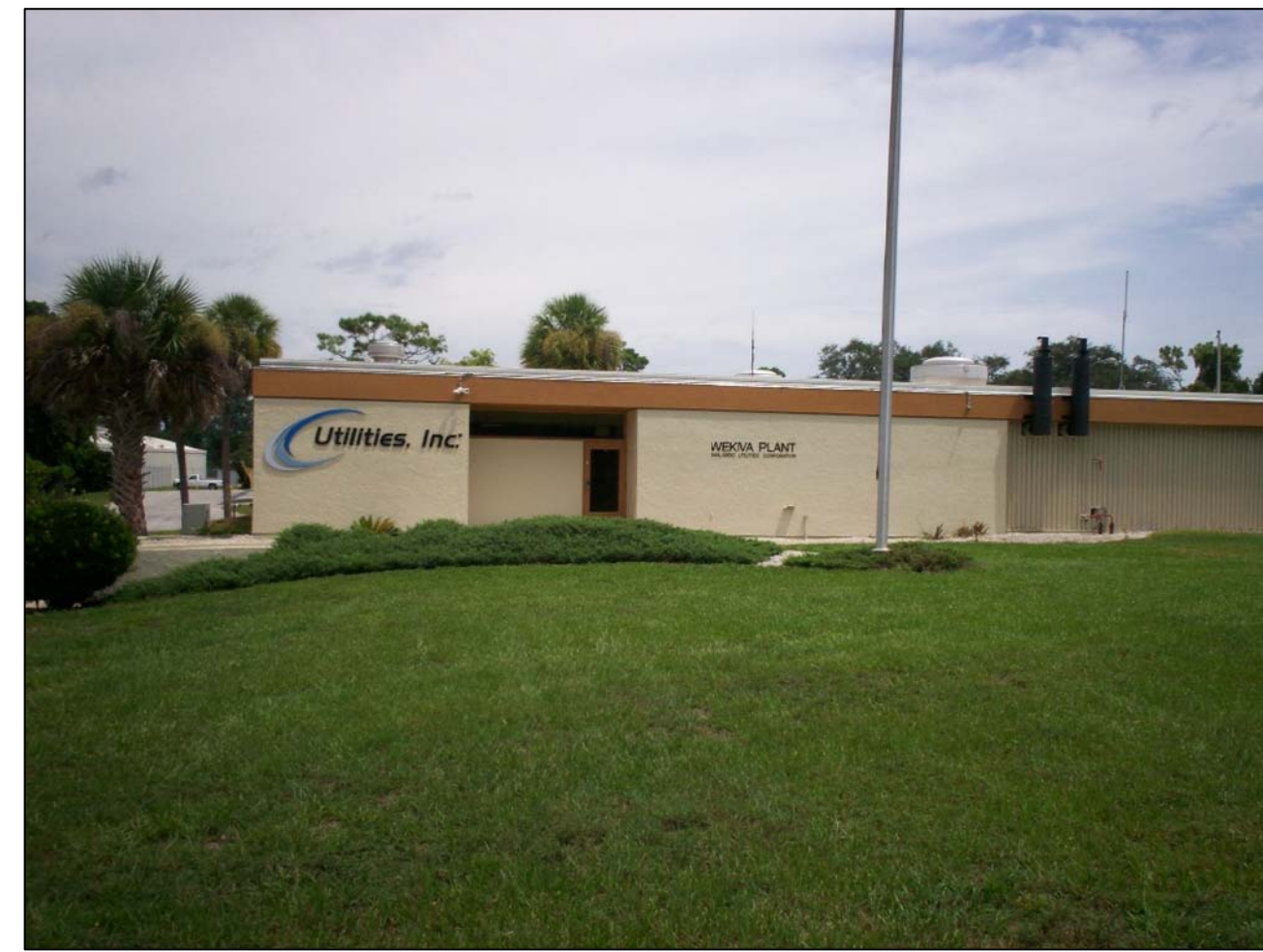
2 SANLANDO - WEKIVA PLANT CONTROL BUILDING
