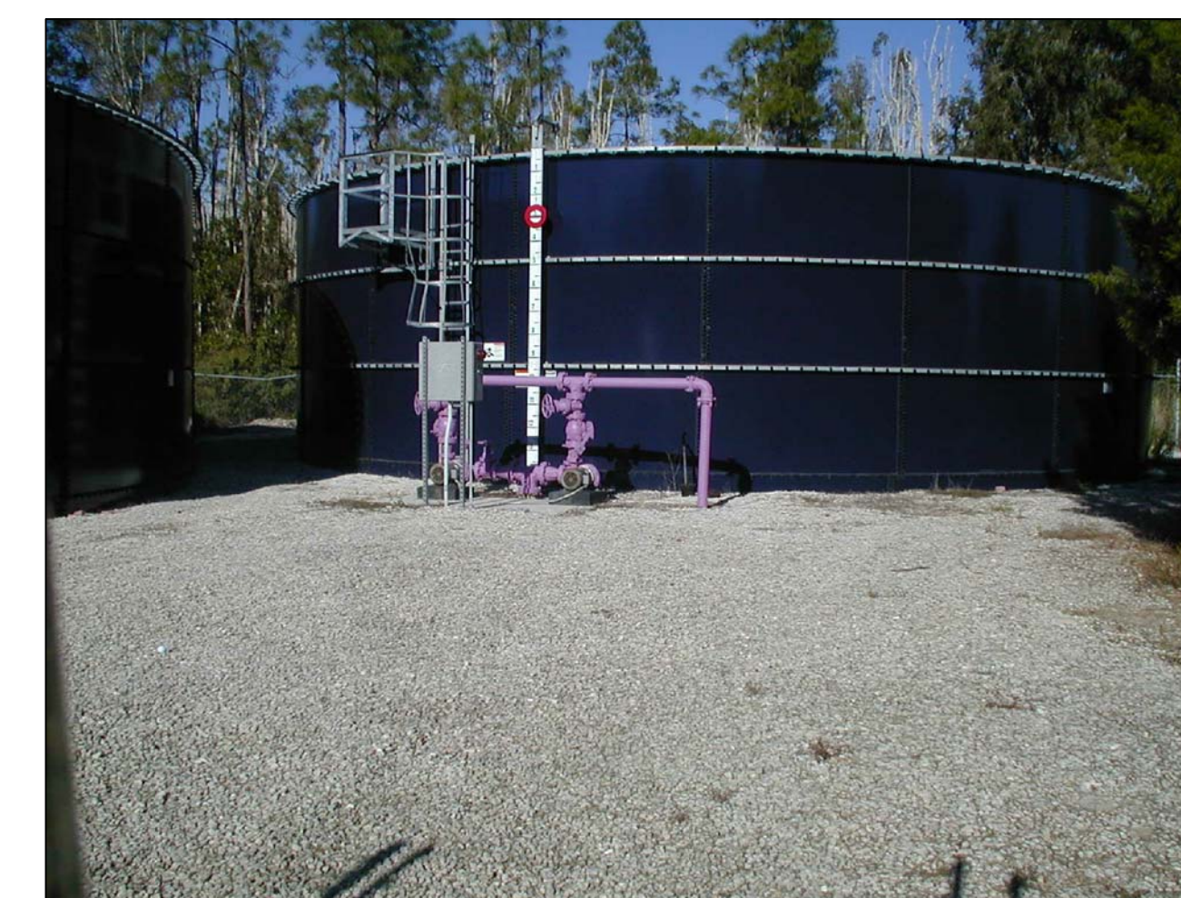
16 CROSS CREEK REUSE PLANT
