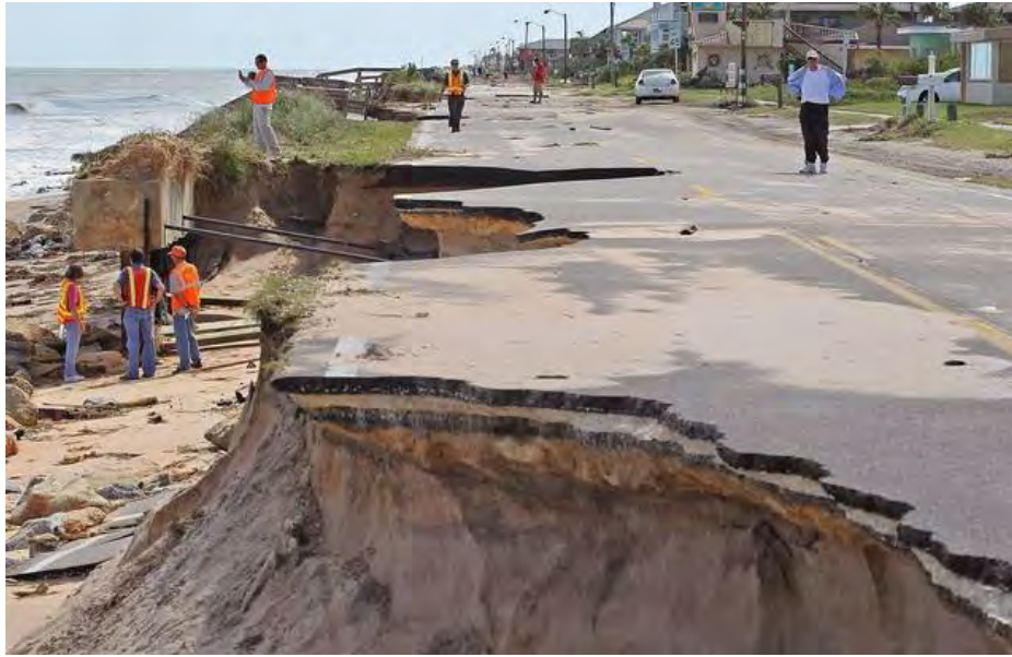
Figure 4: Damage to the AIA in Flagler Beach from beach erosion caused by storm surge and high waves. Courtesy: Miami Herald.
