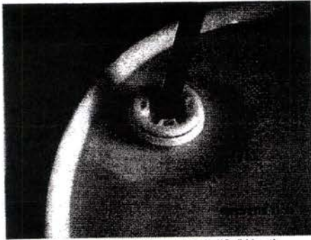
Cross Connection at Barrel Well #2 (West)
