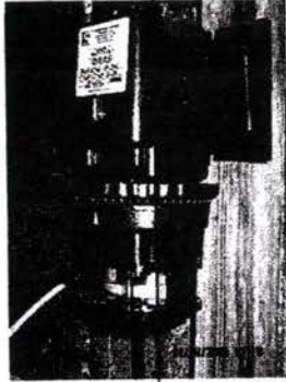
Chlorinator Pump (Well #1) East
