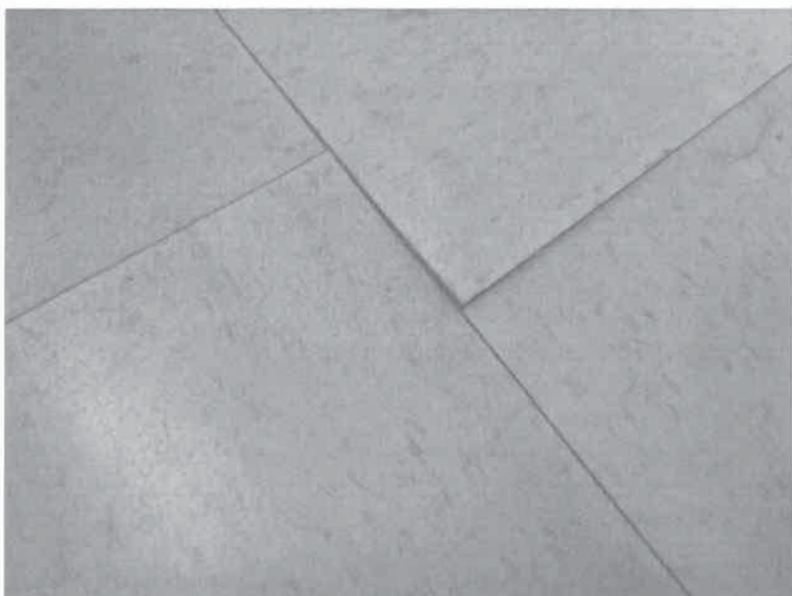
Photo 2. Damaged flooring in one area of elevated moisture levels in floor in reception area
