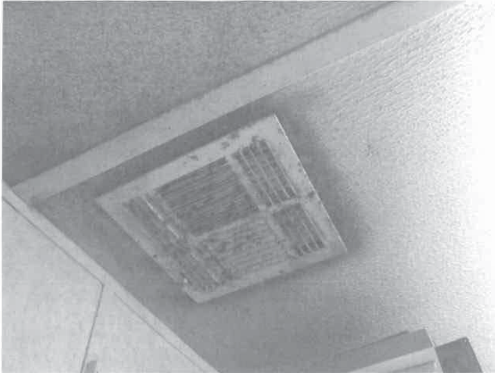
Photo 4. Air conditioning vent in Chris' office with fungal growth. Location of swab surface sample
