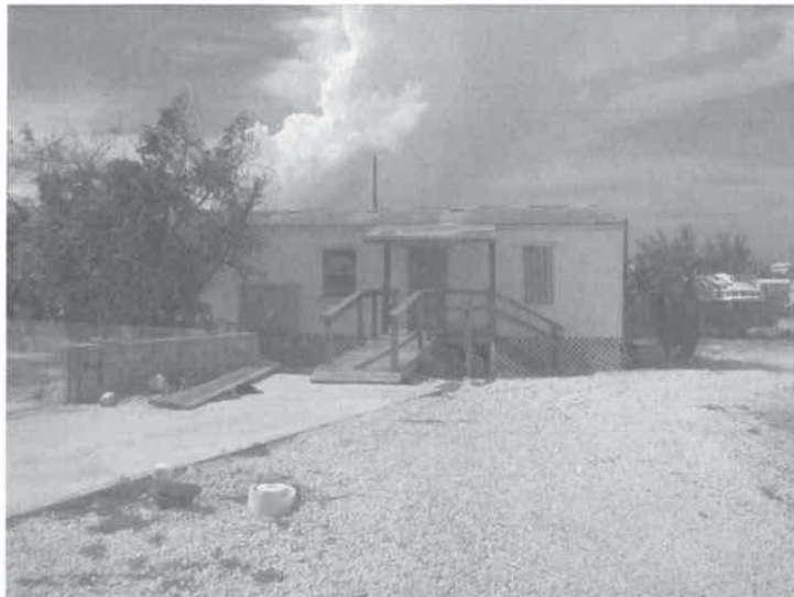
Photo 1. KWRU office building on day of inspection
