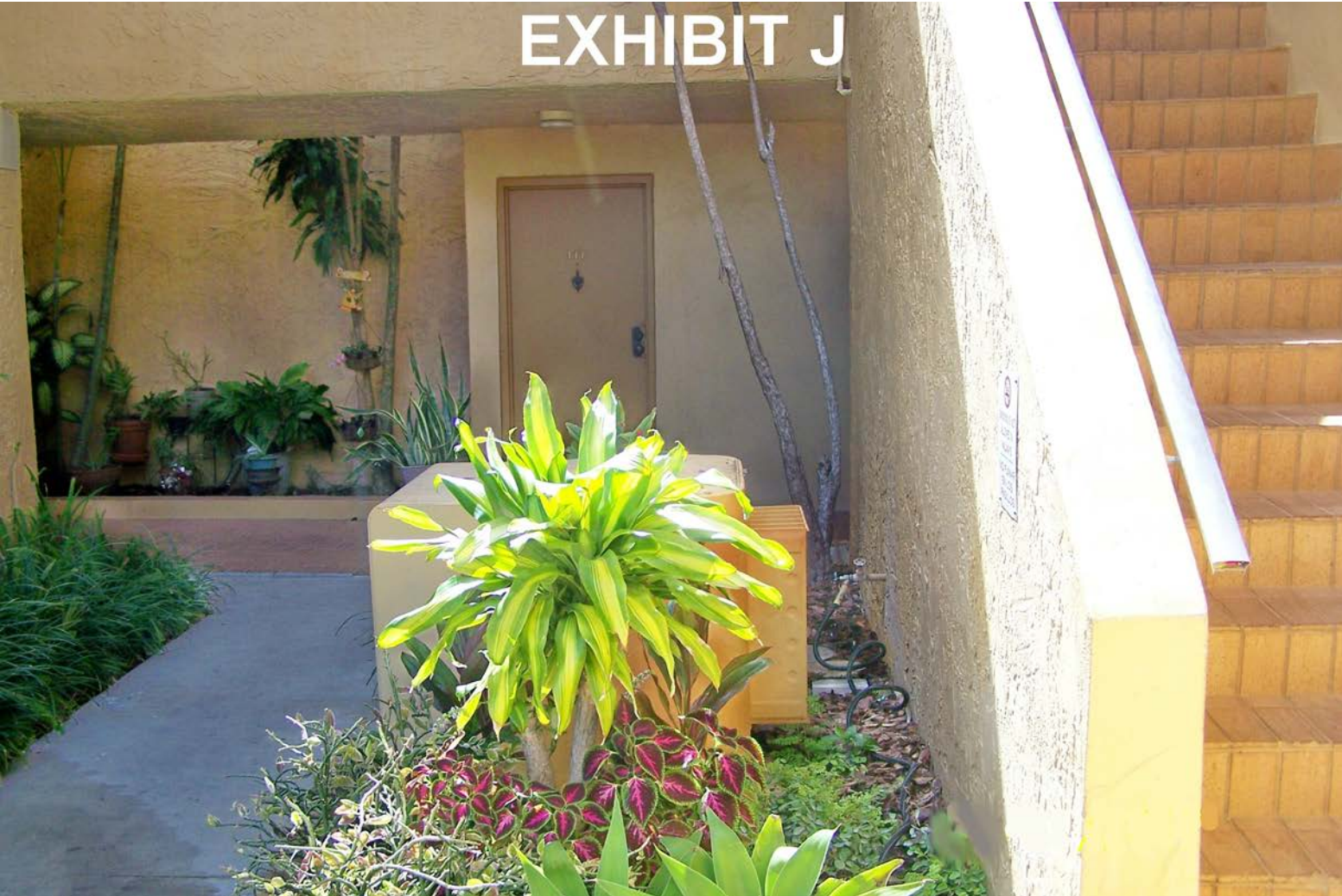
FPL's liquid-filled transformer installed east of Building 9301 in South Winds Condominium
