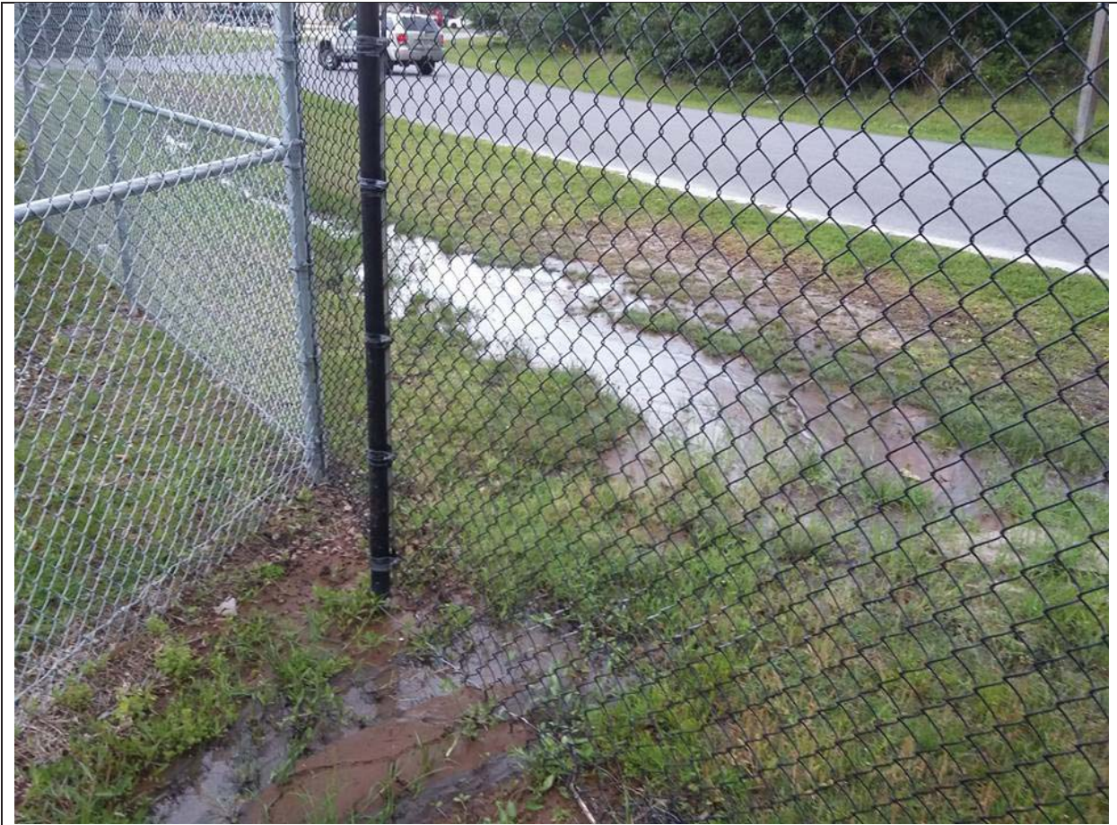
Photo 10 - Pluris water plant, draining from park to street.
