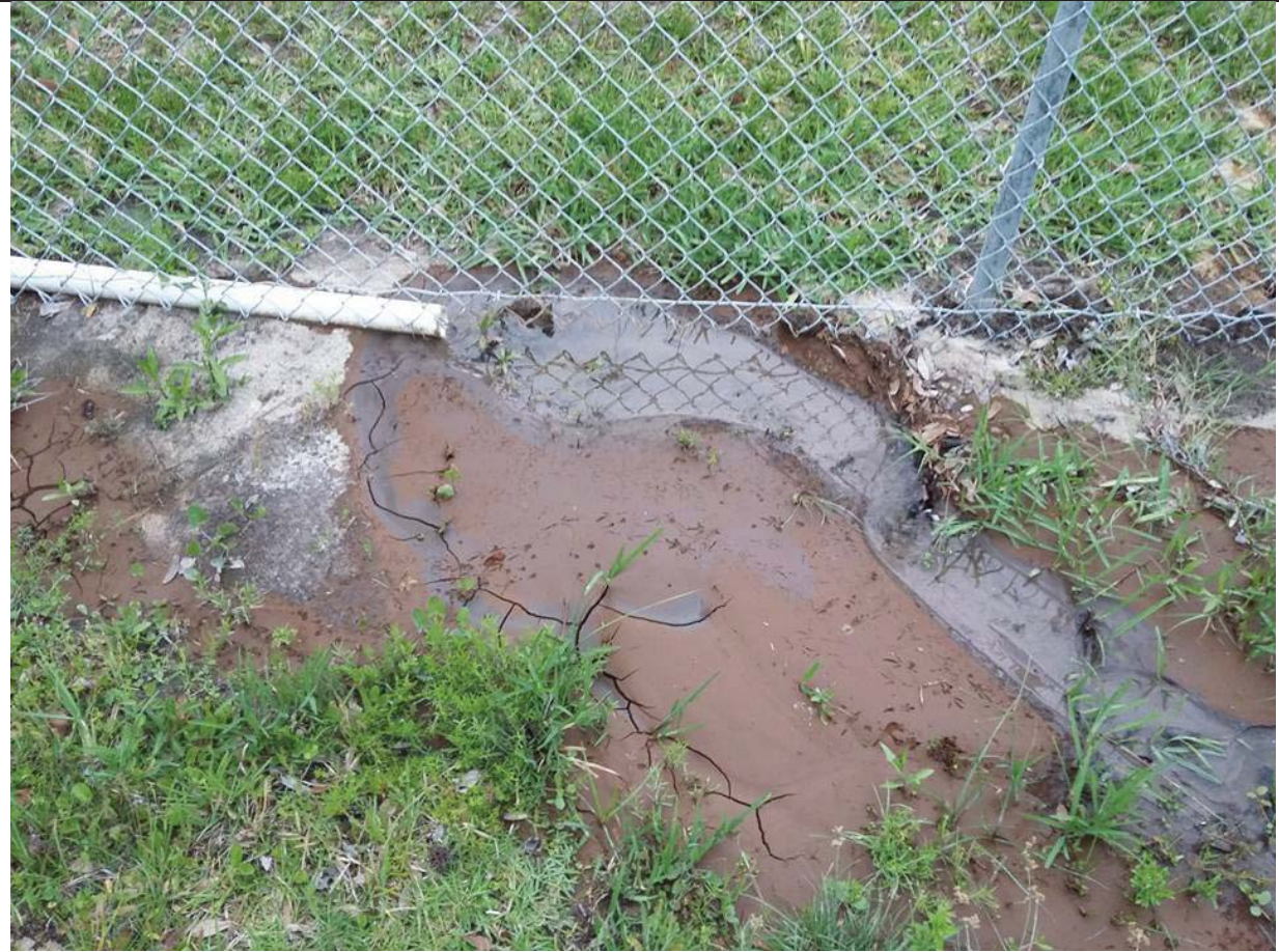
Photo 9 - Pluris water plant, draining into Wedgefield park.
