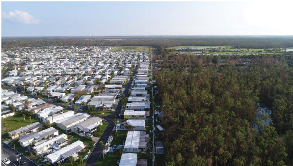
Looking south along feeder.
