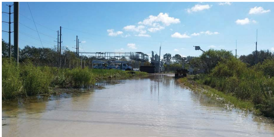
Corkscrew Access Drive
