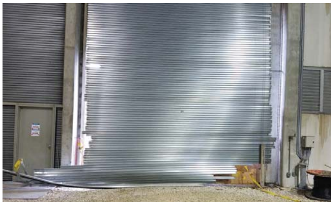
Watkins Substation – Overhead Door
