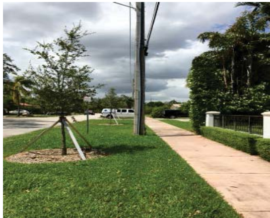
Pictures to the right: Young canopy trees (i.e. oak) and palms planted in the wrong place and will impact facilities in the future
