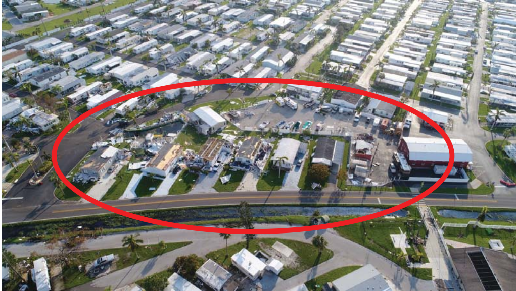
Area of concentrated damage, looking west.
