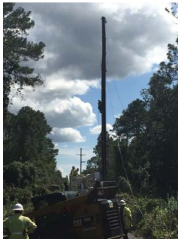
Pole Replacement of Structure 75G3 (115KV line in North area)
