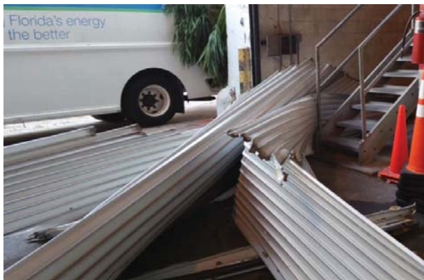
Watkins Substation – Overhead Door
