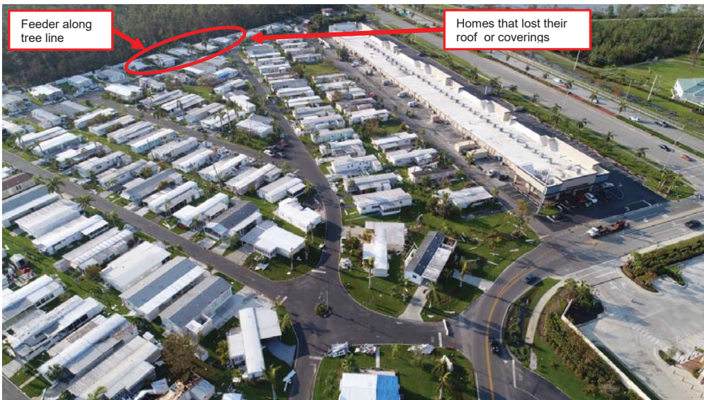
Looking northwest through the trailer park toward the feeder
