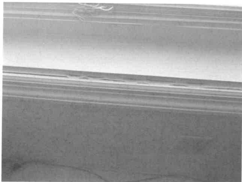
Photo 24. Damage to window frame in Kaitlin's office
