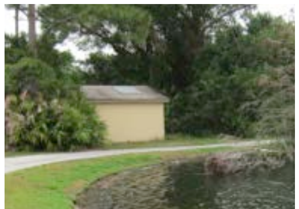
Figure-2 shows the prefabricated pumping station on the left and Figure-3, a similar installation at the Sandridge Golf Course, below. Our installation will match the existing toilets.
