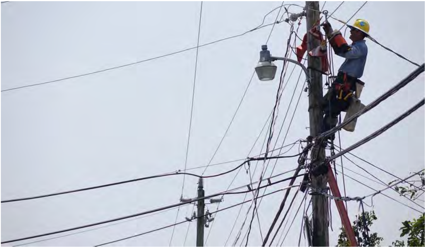
A lineman working with Florida Power and Light connects residence in Oakland Park after 2017's Hurricane Irma. (JOE CAVARETTA / Sun Sentinel)
