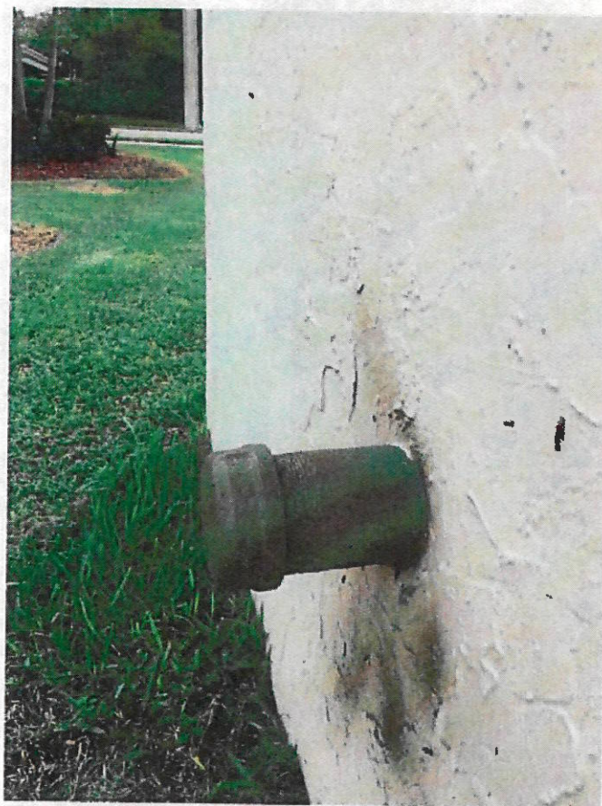
FIGURE 6. WELL #3 FLUSH LINE CAP TIGHTENED, WIIRE BRUSHED, AND ANTI CORROSION COATED.
