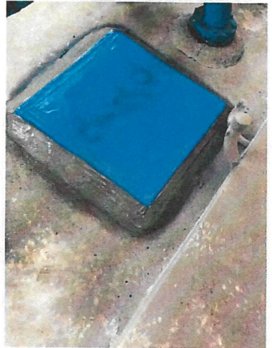
FIGURE 2. POSITION FOR FUTURE BWT #2 SEALED.
