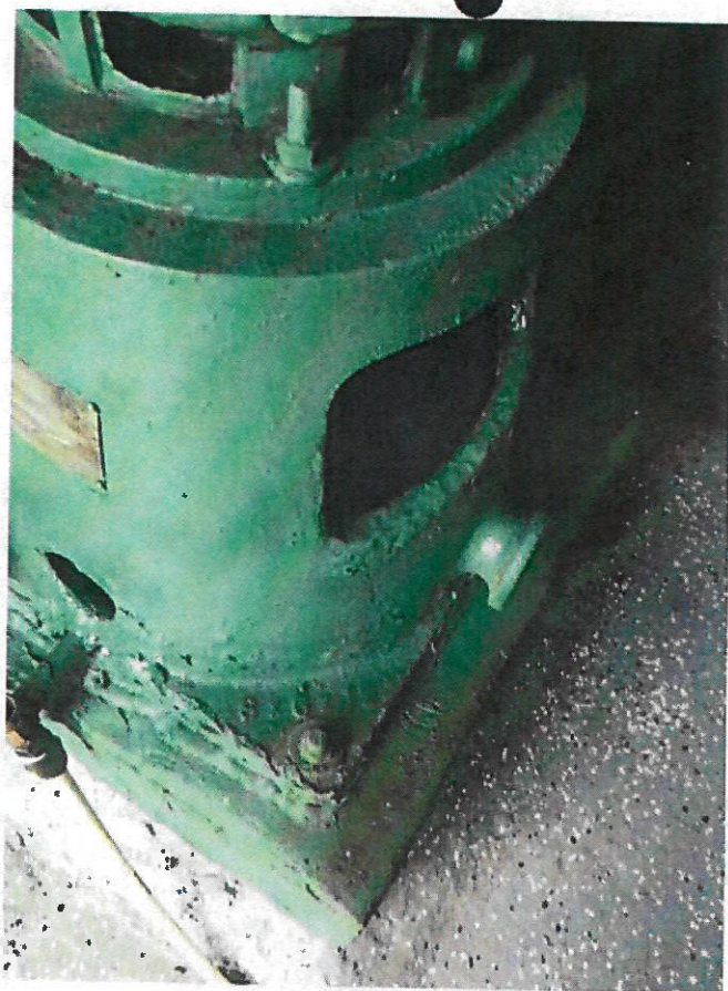
FIGURE 5. WELL #3 CORROSION AREAS WIRE BRUSHED, ANTI CORROSION COATED
