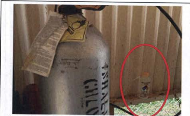
Ammonia bottle must be properly labeled.
