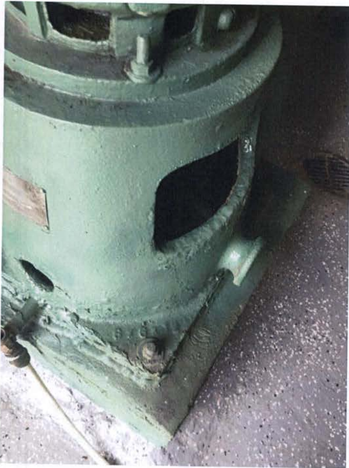
FIGURE 7. WELL #3 CORROSION AREAS WIRE BRUSHED, ANTI CORROSION COATED
