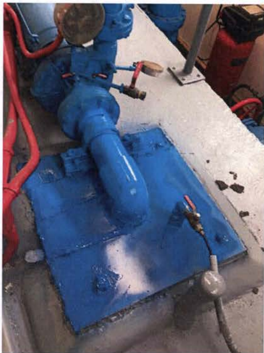
FIGURE 1. ALUMINUM PLATE SEALED OVER CLEARWELL ALL SEAMS/OPENINGS AND CAULKED WITH SILICONE.
