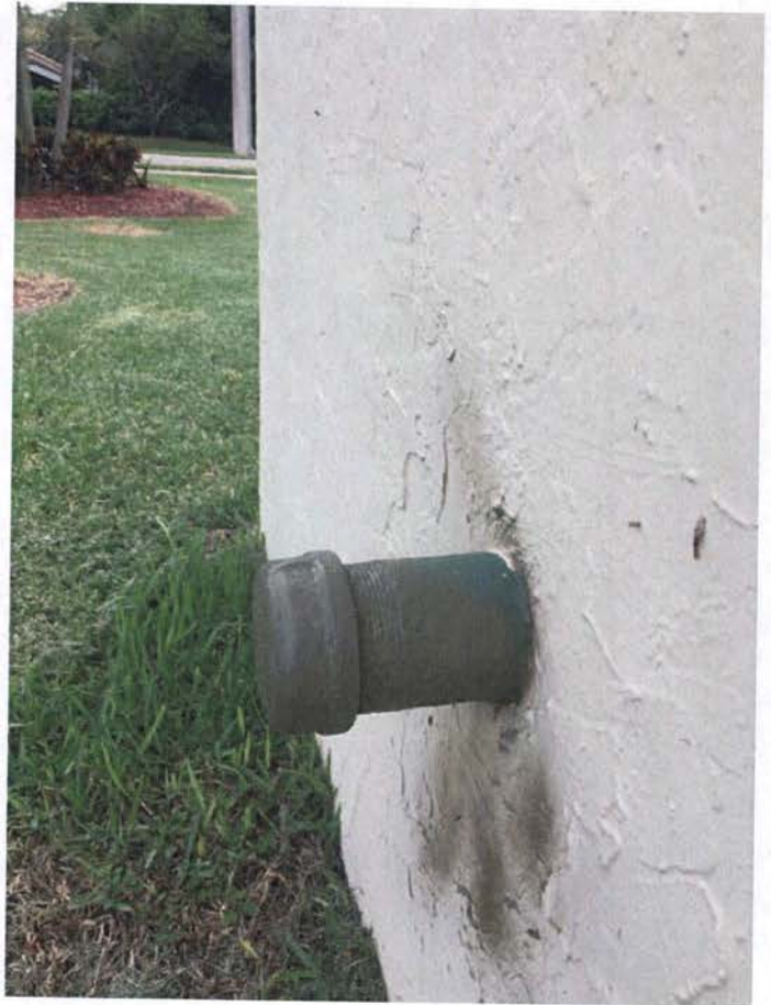
FIGURE 8. WELL #3 FLUSH LINE CAP TIGHTENED, WIIRE BRUSHED, AND ANTI CORROSION COATED.
