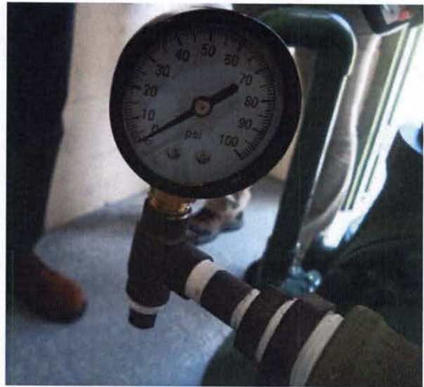
Figure 6. New pressure gauge installed at well#2.
