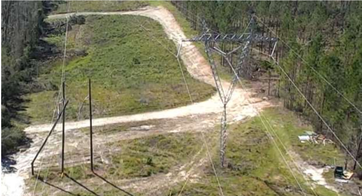
FIGURE 8 – GUYED Y TOWER
