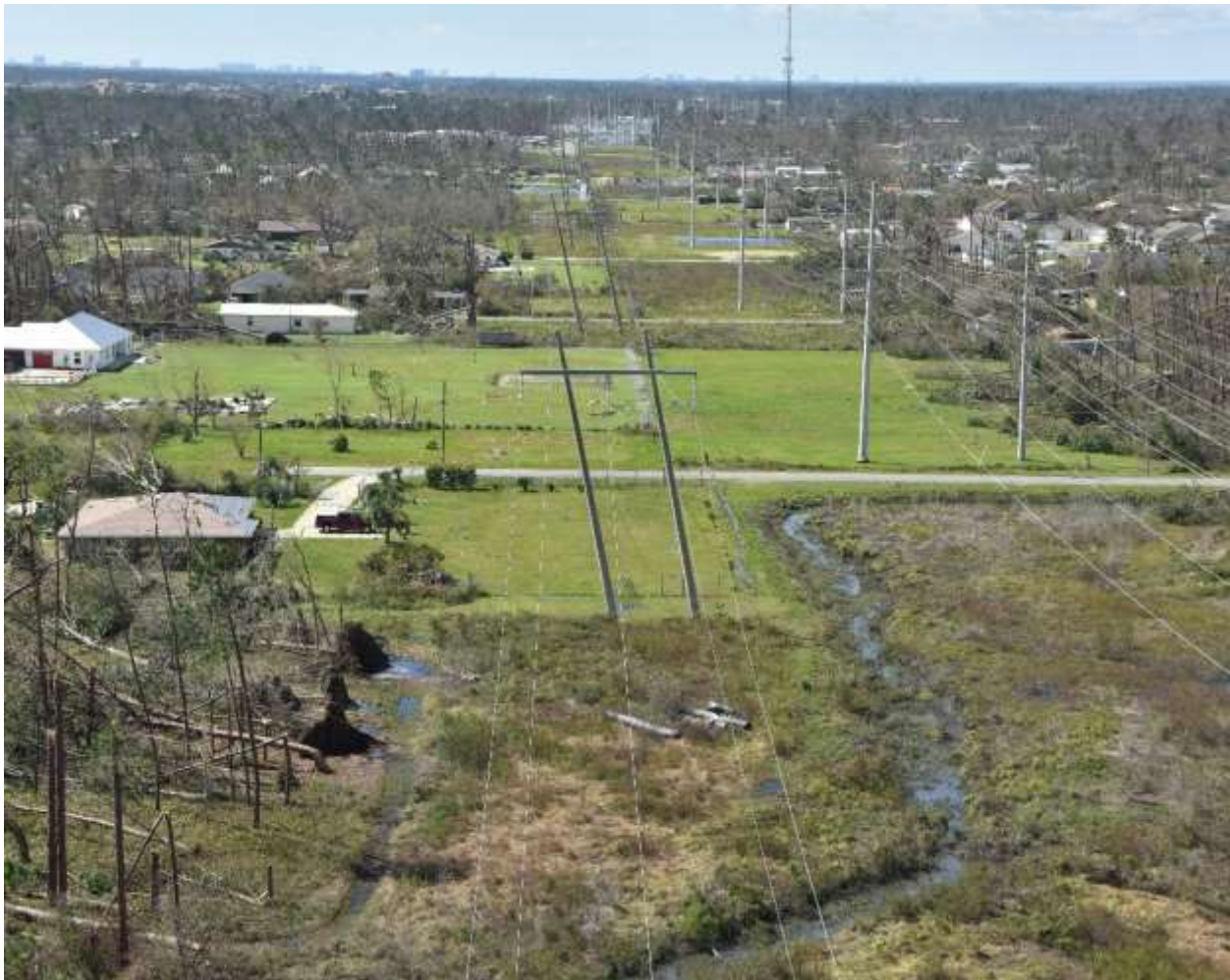
FIGURE 3 – CONCRETE WITH AND WITHOUT STORM GUYS
