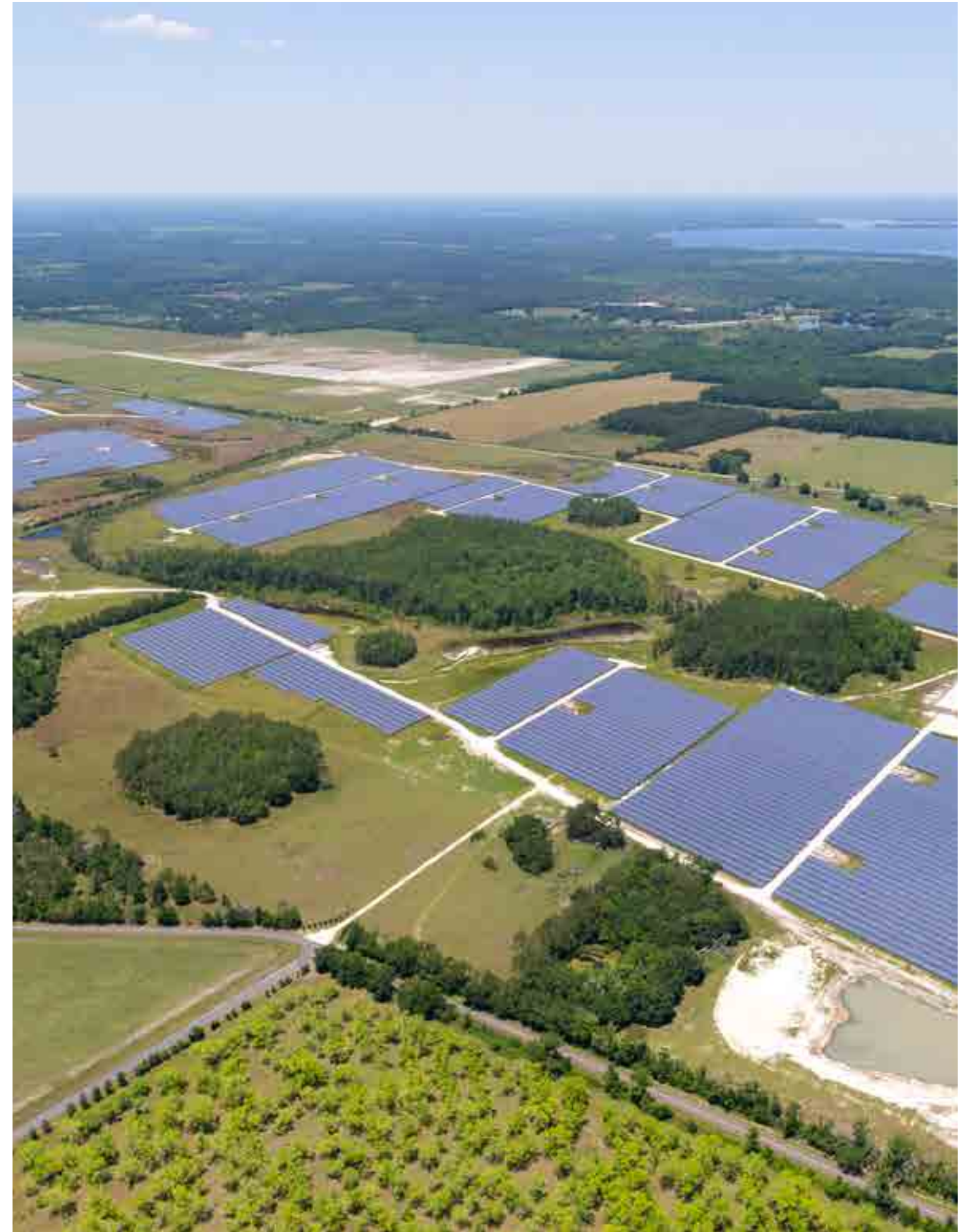
FPL Horizon Solar Energy Center is situated on the border of Alachua and Putnam counties
