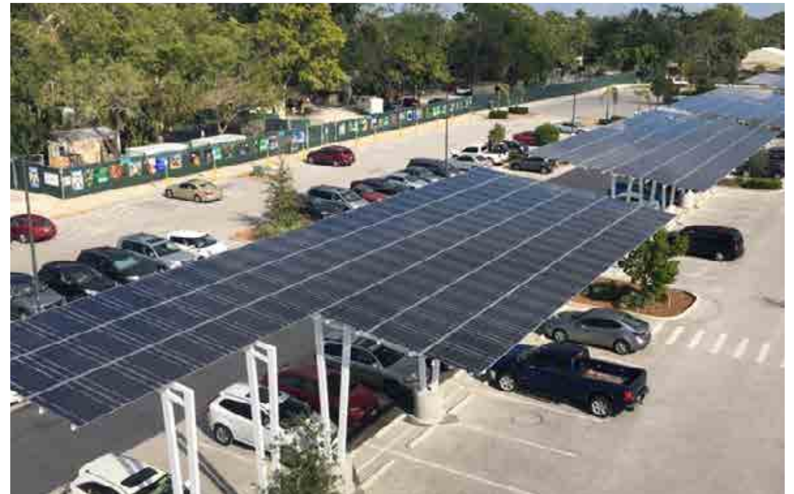
Opposite and this page: Naples Zoo at Caribbean Gardens, Collier County, is home to a ~200 kilowatt solar canopy that also provides shaded parking for visitors
