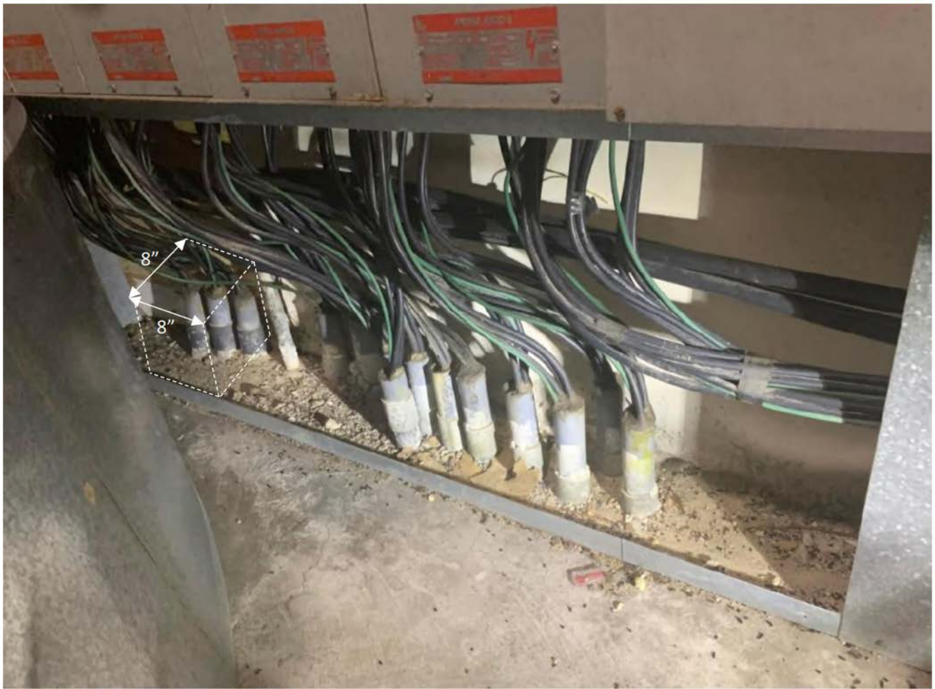
Photo 2: Existing inside wire enclosure
