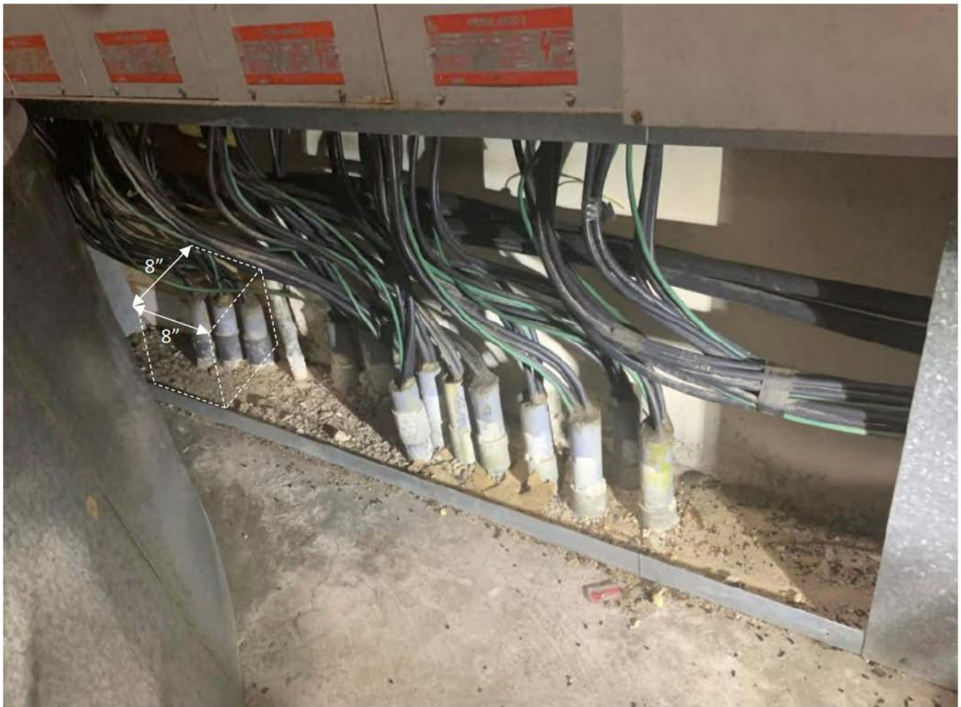
Photo 2: Existing inside wire enclosure
