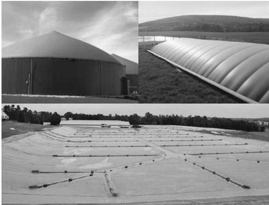
Figure 7: Complete-Mix Tank (Top Left), Plug Flow (Top Right), and Complete-Mix Lagoon (Bottom) Anaerobic Digesters
