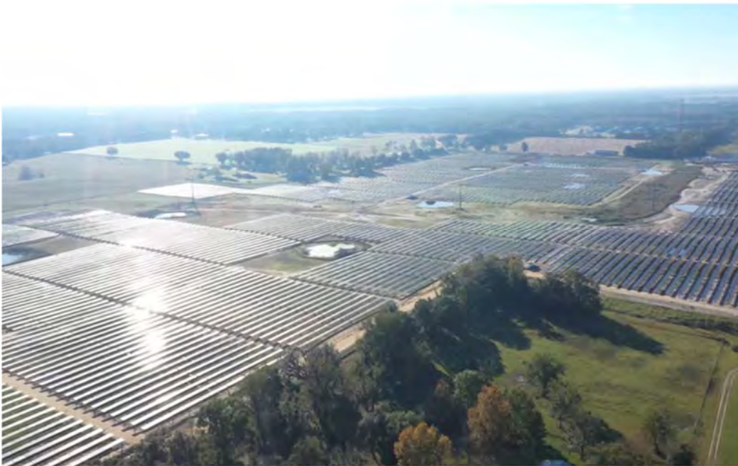
FIGURE 3.7 Trenton Solar Site
