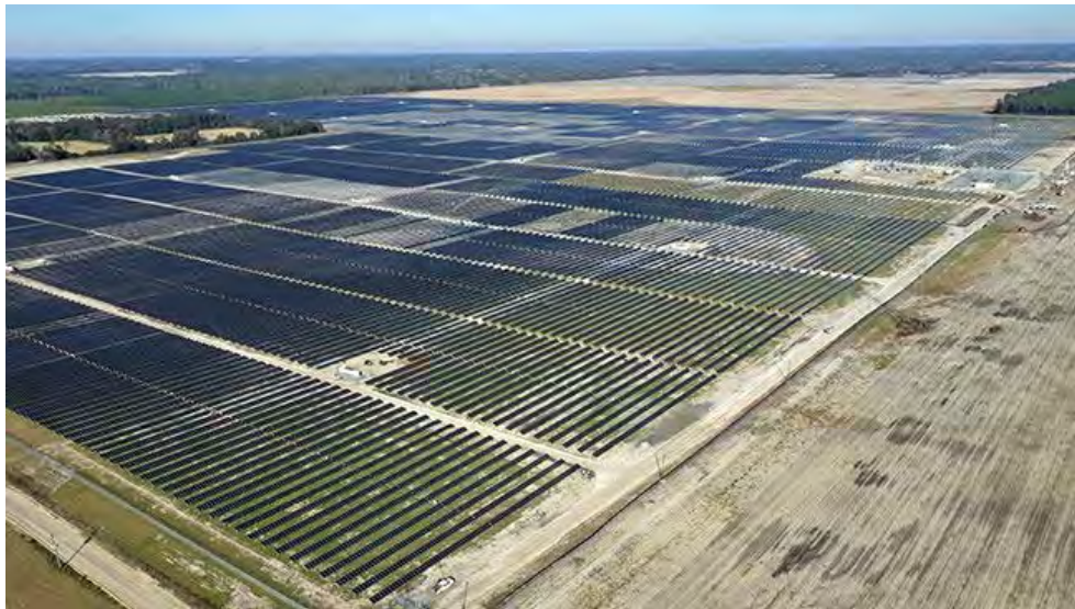
FIGURE 3.5 Hamilton Solar Site
