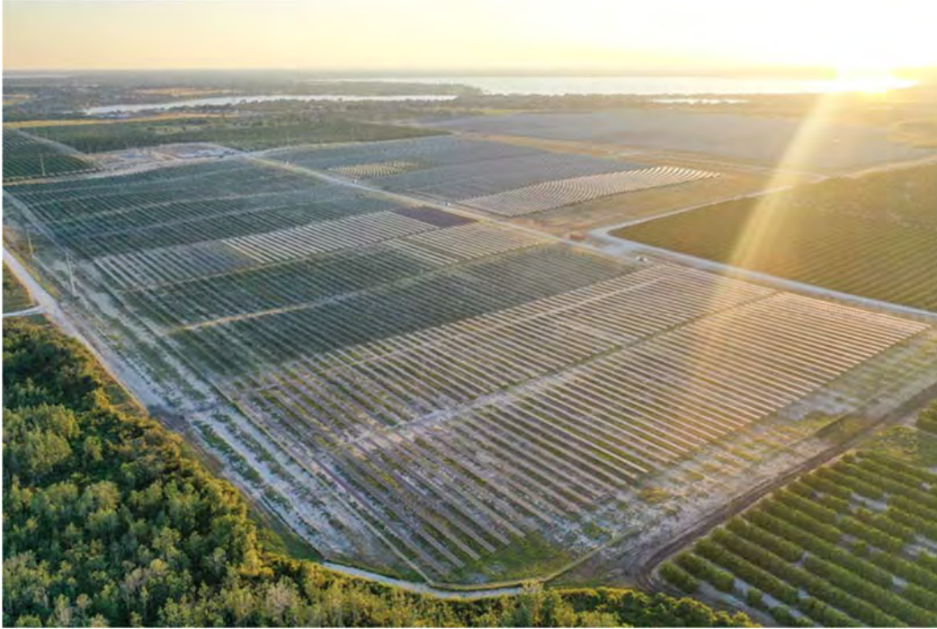
FIGURE 3.6 Lake Placid Solar Site
