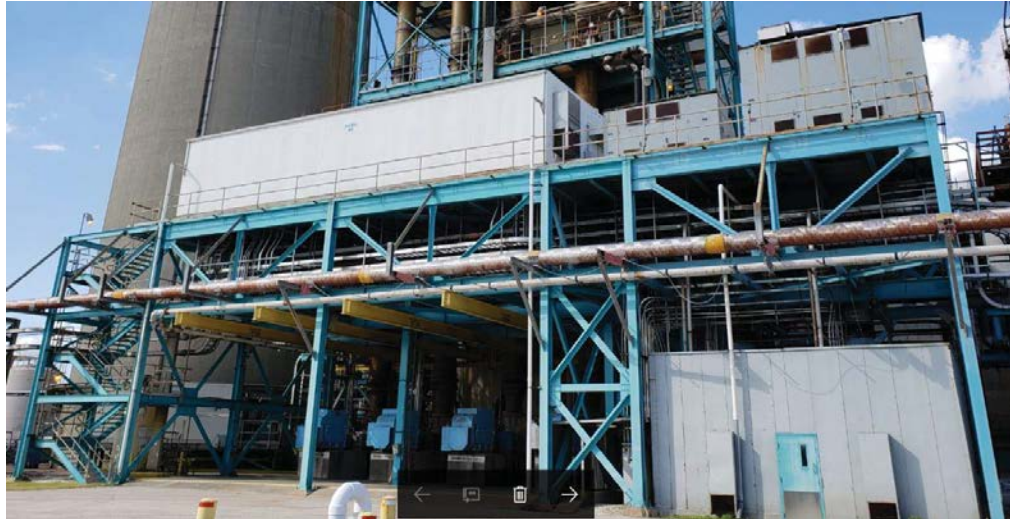
Figure 4 – Units 1 and 2 WFGD Electrical Building-to remain
