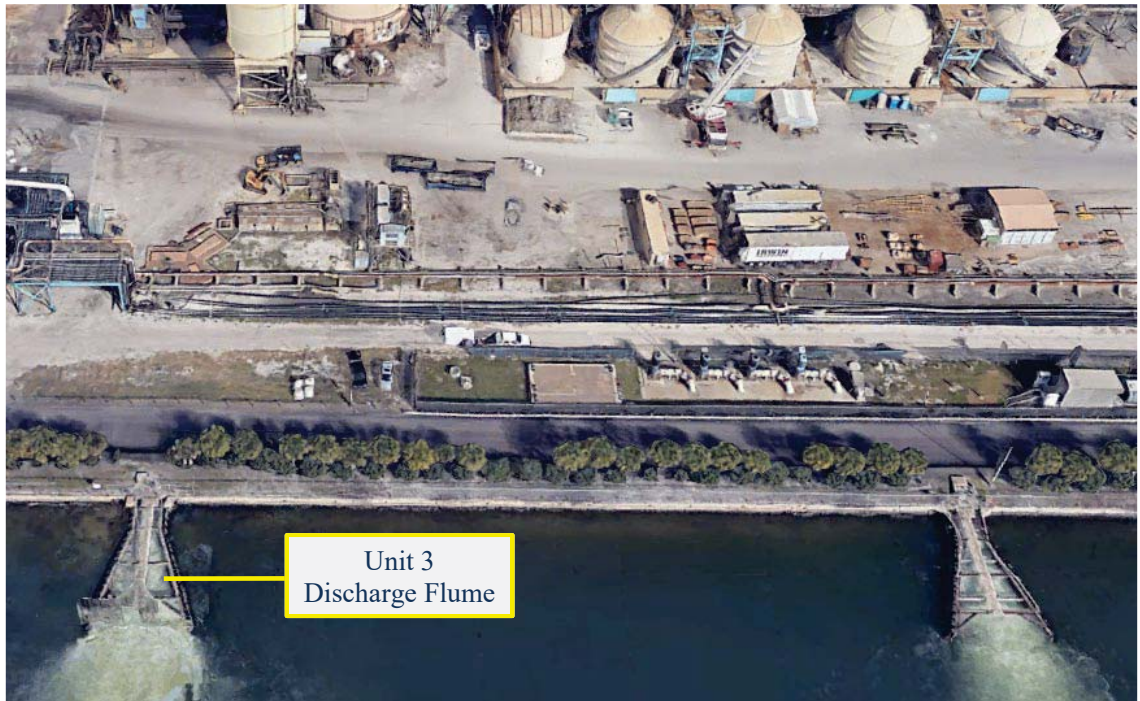
Figure 5 – Unit 3 and 4 Circulation Water Discharge Area
