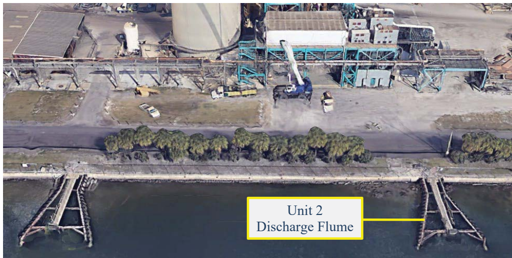
Figure 5 – Unit 1 and 2 Circulation Water Discharge Area
