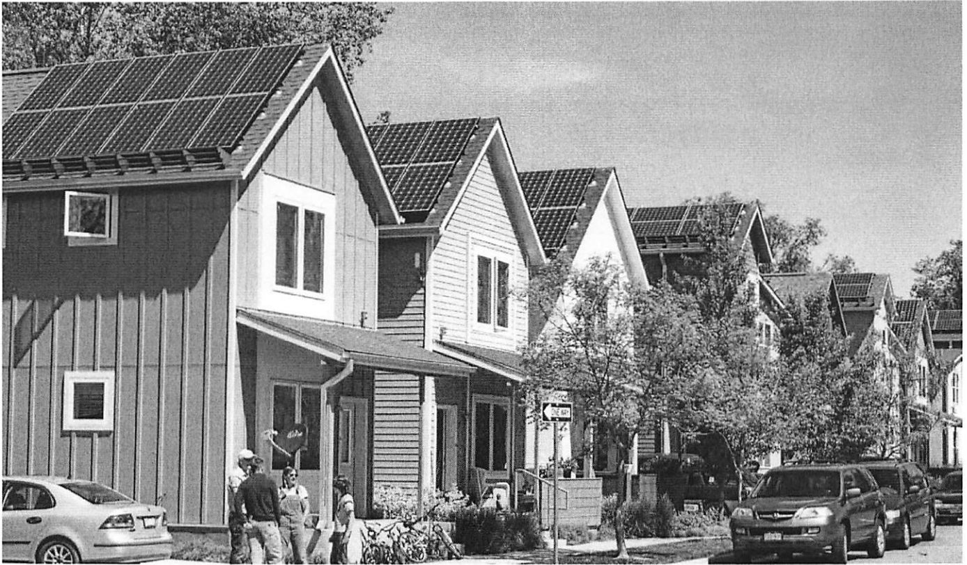
Photo by Dennis Schroeder via National Renewable Energy Laboratory, CC BY-NC-ND 2.0.
