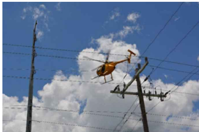
DETAIL F - HELICOPTER WIRE PULL
