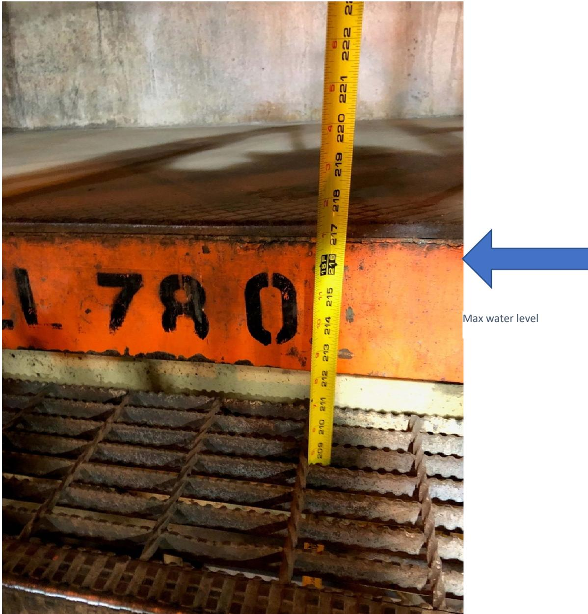
**Water level was 18ft above general sub-basement elevation in unit 6&7 with some areas deeper with equipment wells**
