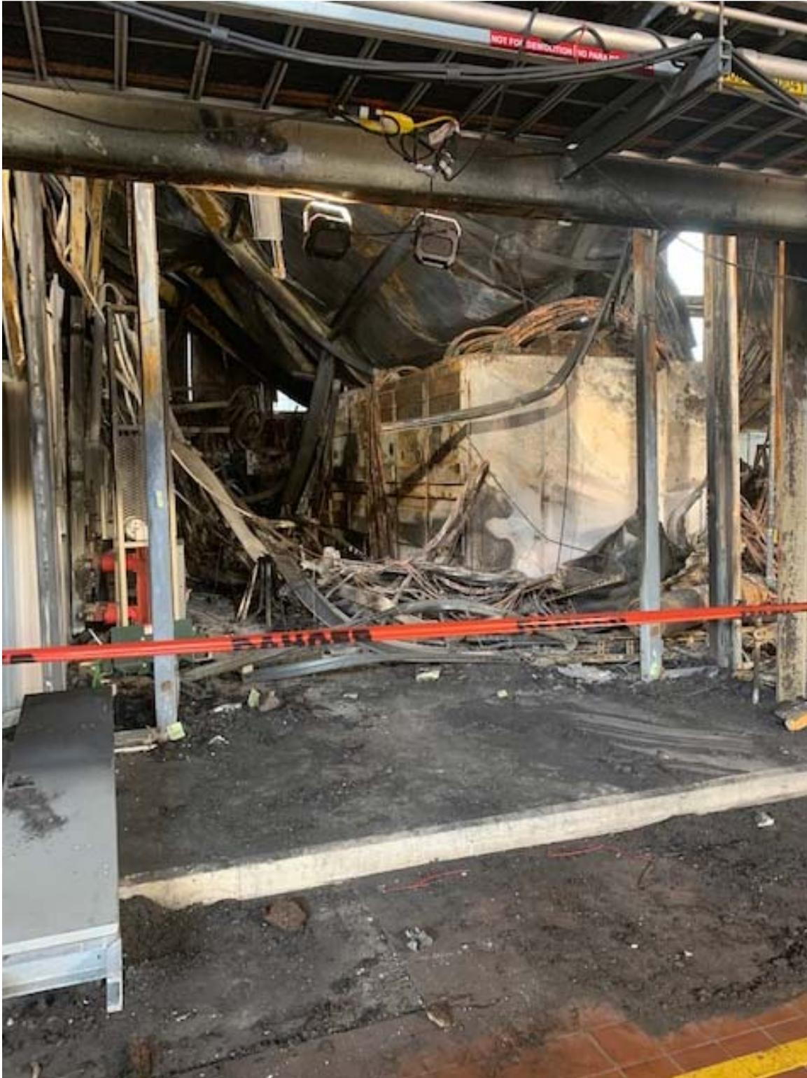
**6C/7C 4160V AC switchgear and surrounding building. Fire damage**
