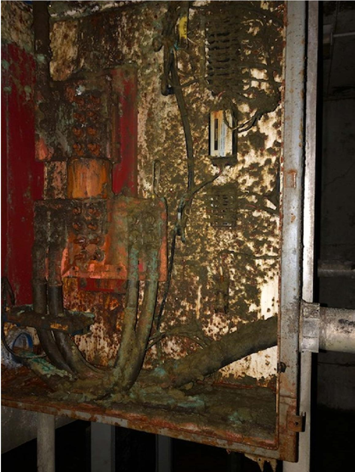
Example of a 125 VDC electrical panel after dewatering. Corrosion present.
