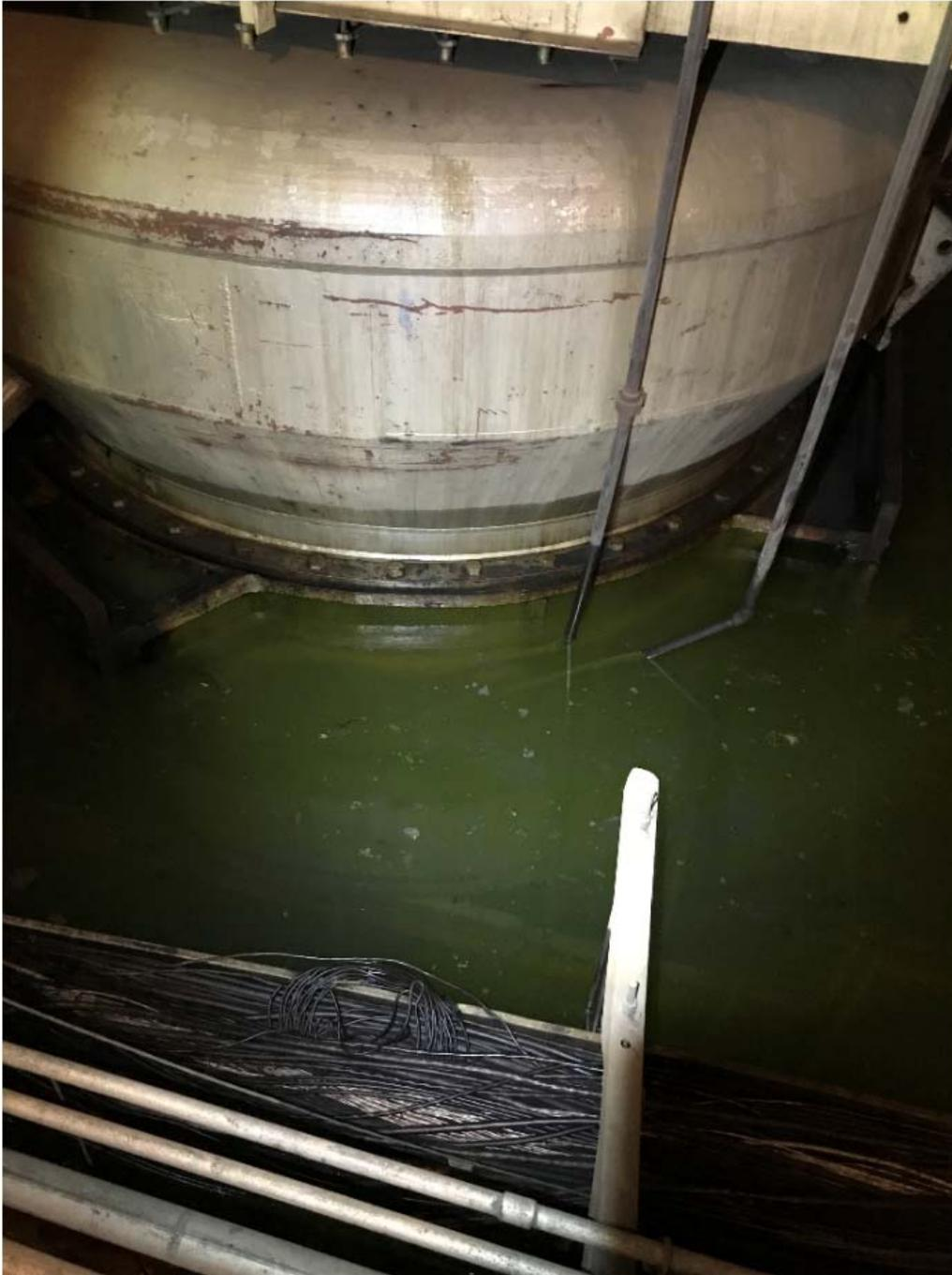
**Flooded coal pulverizer, picture of 6A under 18 ft of water**
