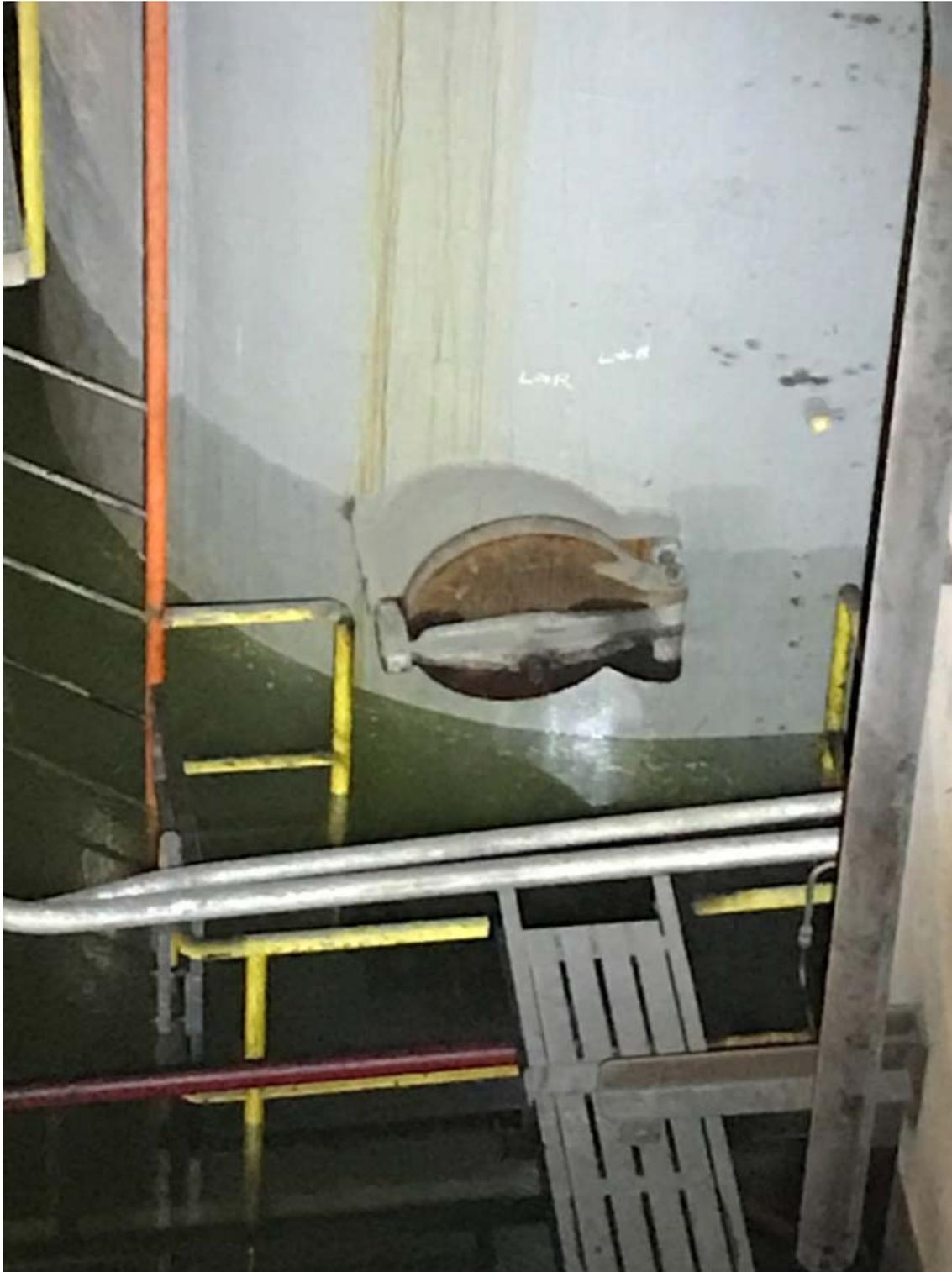
Unit 6 condenser waterbox door. Note water line at approximately 18 ft from general sub-basement floor
