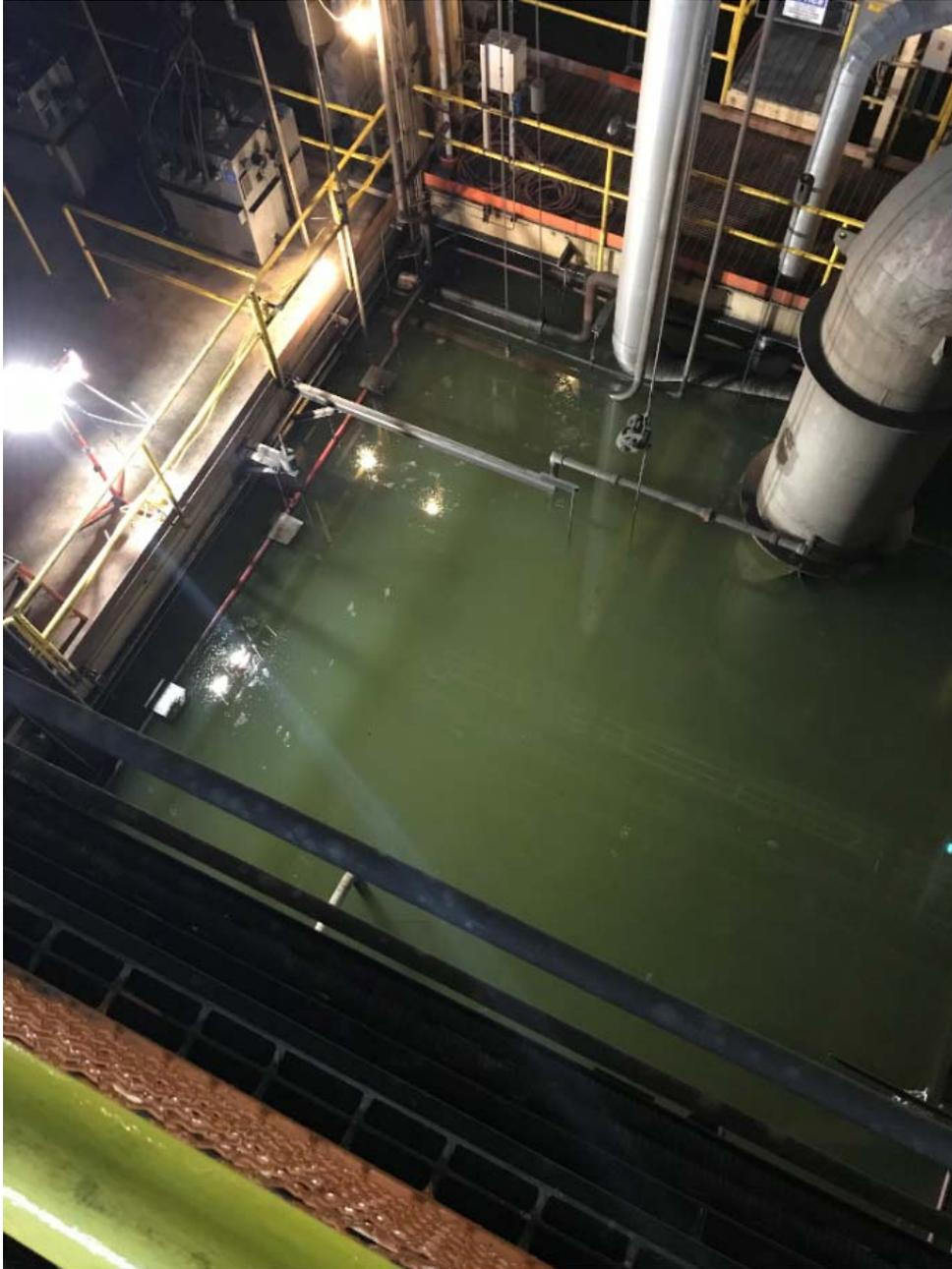
**Boiler Feed Pump turbine exhaust, boiler feed pump turbine and pump submerged below**
